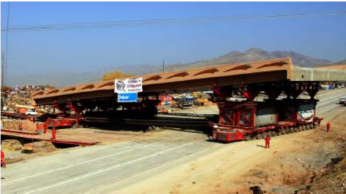
Figure 6 – New Span on SPMTs: 4500 South over I-215
