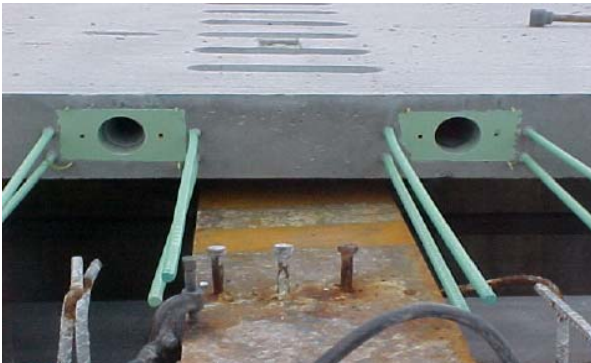
Figure 2 – Post-Tensioned Deck: I-215 over 3900 South
