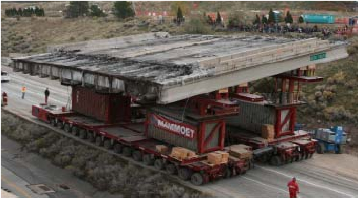
Figure 5 – Removal with SPMTs: 4500 S over I-215
