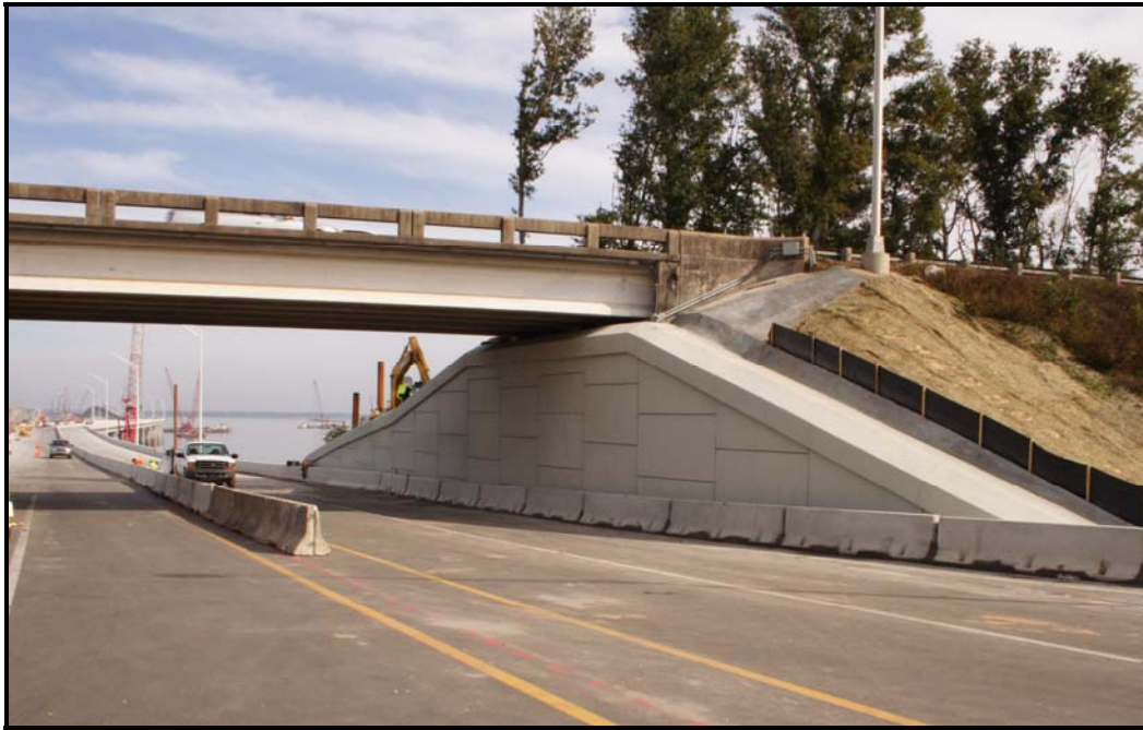
Figure 3 – Retaining Wall Under Scenic Highway
