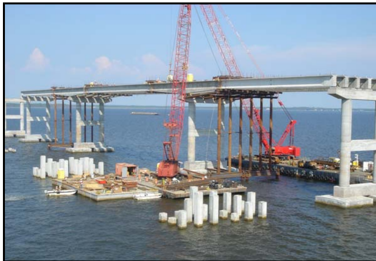
Figure 4 – Spliced Girder Erection
