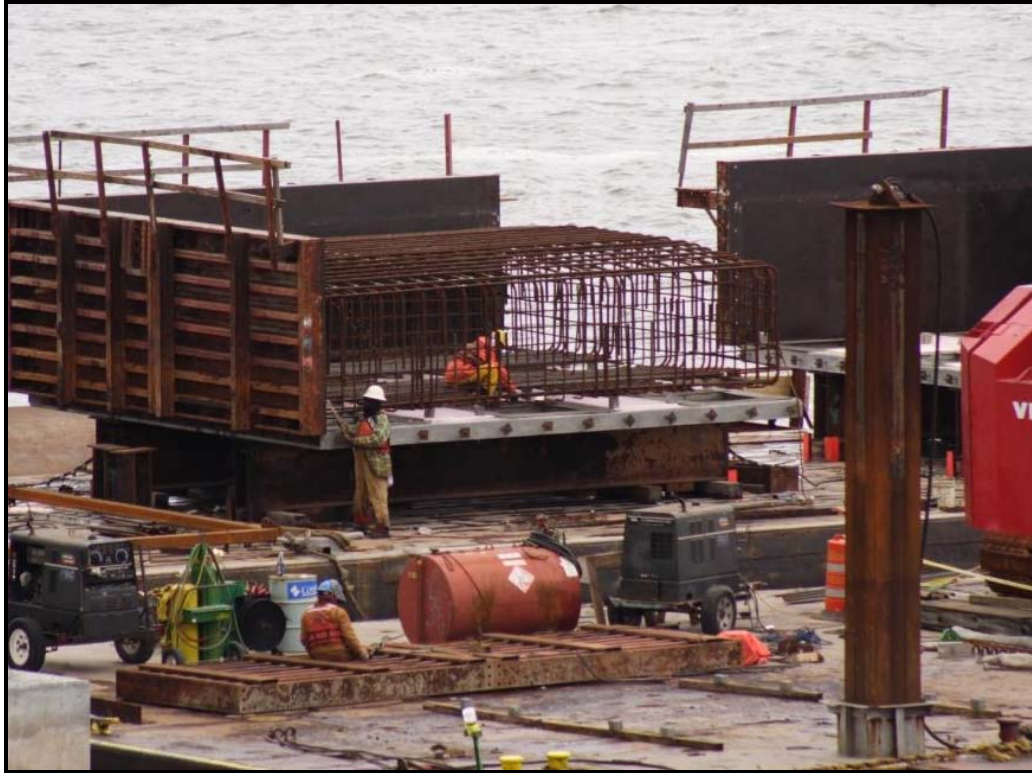
Figure 14 – CIP Footing Preparations
