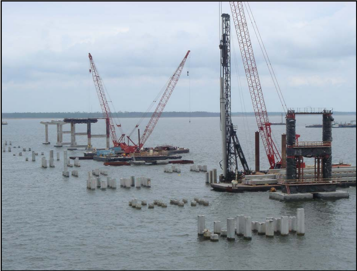
Figure 13 – Pile Driving
