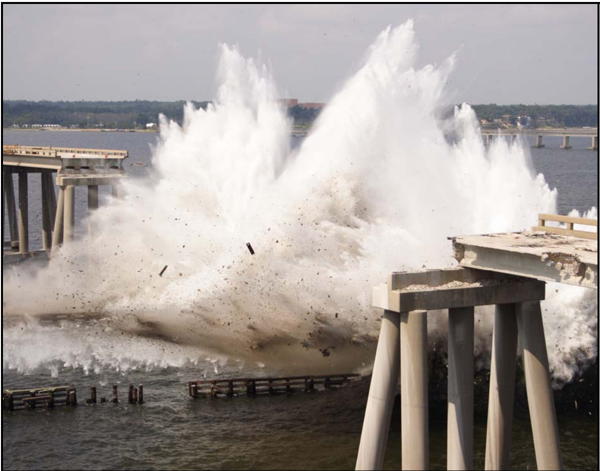
Figure 19 – Demolition of Existing Bridges
