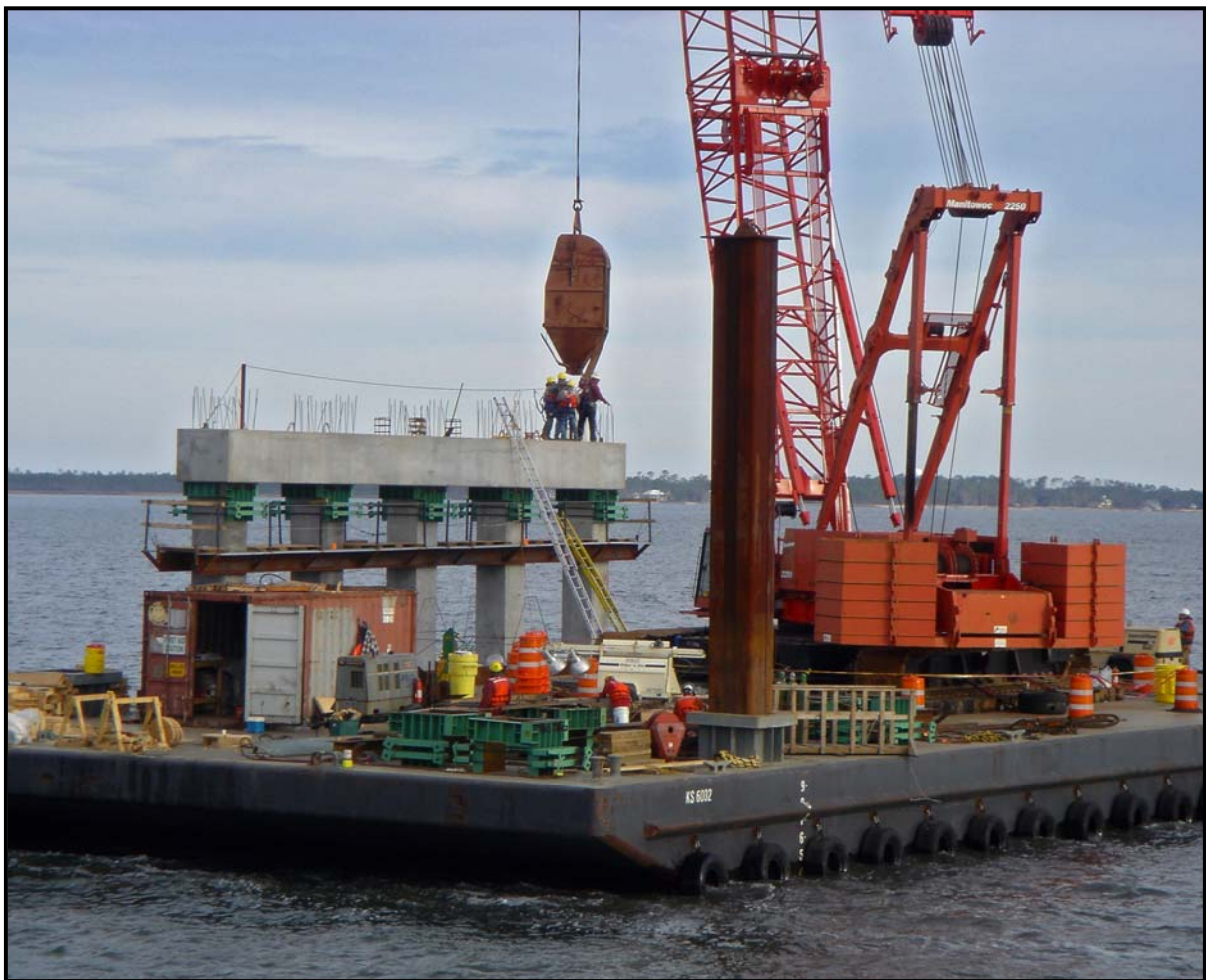
Figure 6 – CIP Pile Cap Connection
