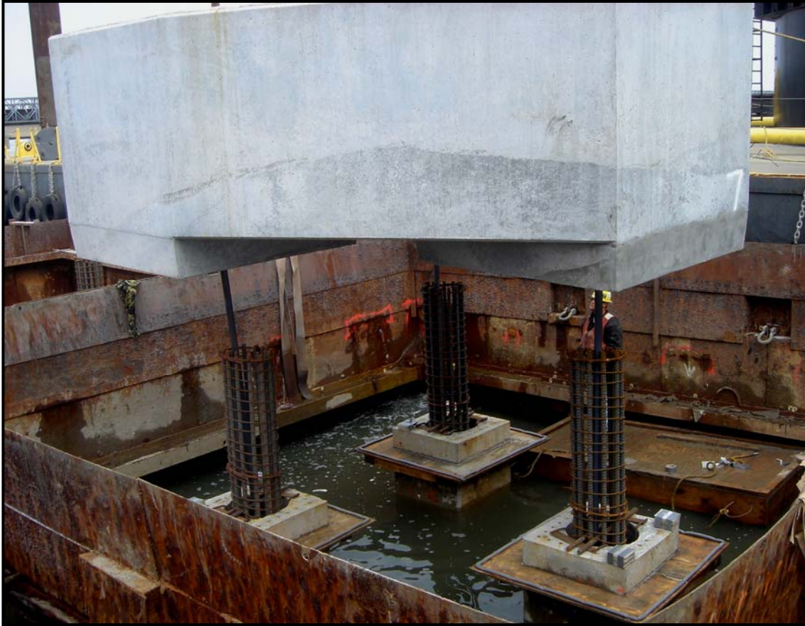
Figure 12 – Precast Pile Footing
