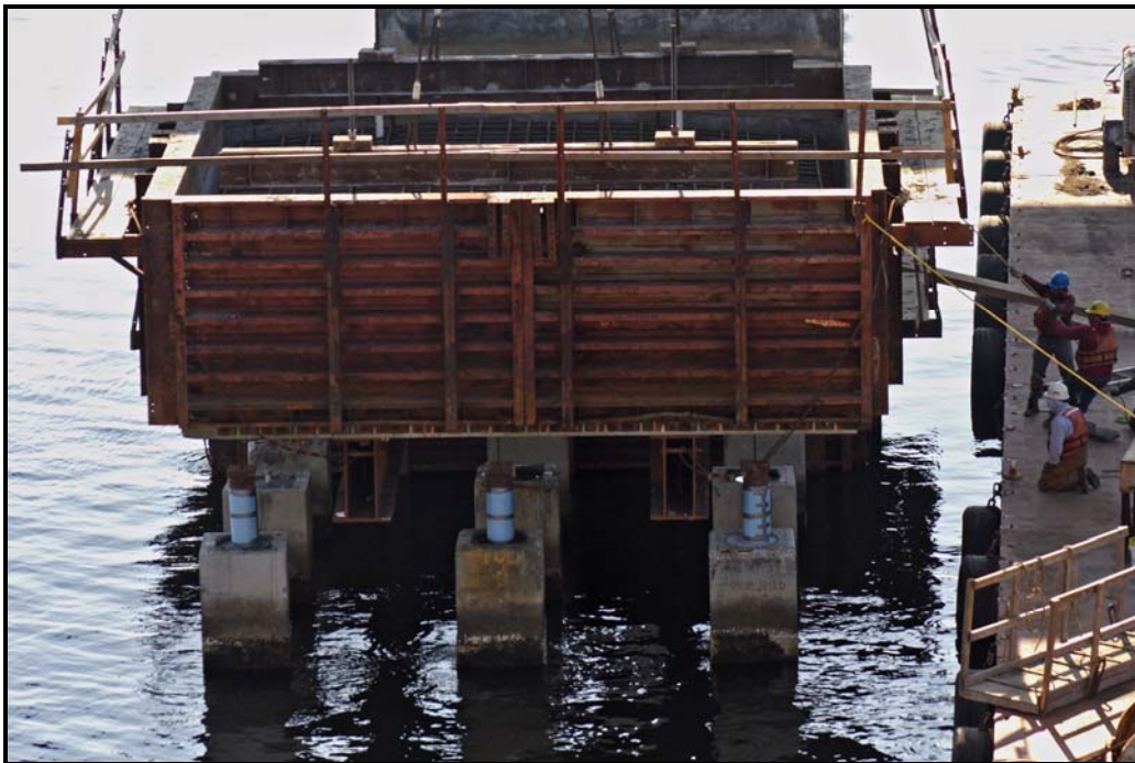
Figure 15 – CIP Footing, Formwork, and Rebar Cage Set in Place
