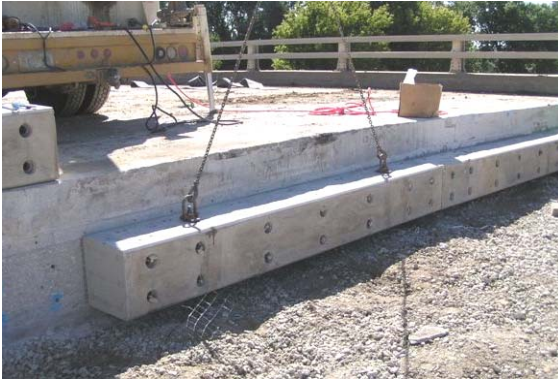
Figure 25. Field implementation of precast paving notch system on bridge VALUE OF TESTING AND EVALUATION
