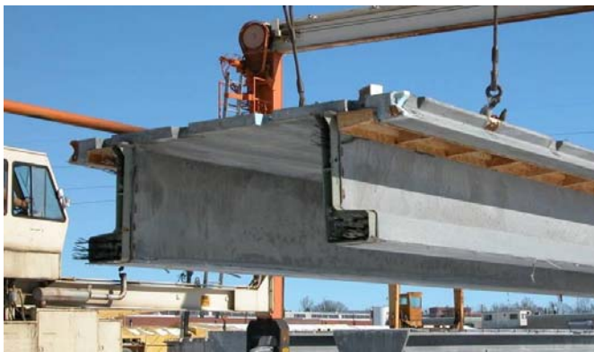
Figure 7. First generation Pi girder
