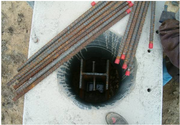
a. Setting precast abutment
