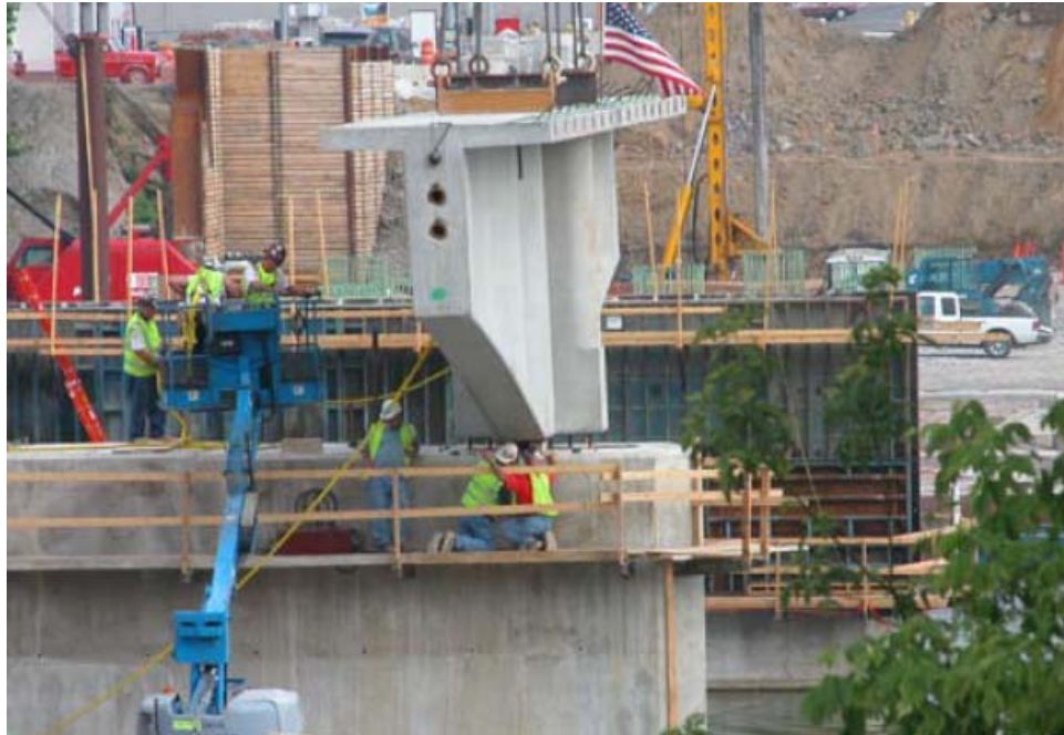
Fig. 2 Pier Segment of a Spliced-Deck Bulb-tee Girder Bridge (Perry Street Bridge, Ohio)
