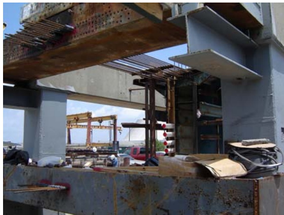
Fig. 10 Compression frame for haunched girder pre-tensioning
