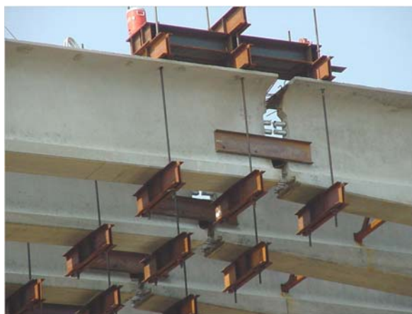
Fig. 13 Common beam hanger or “strongback” concept
