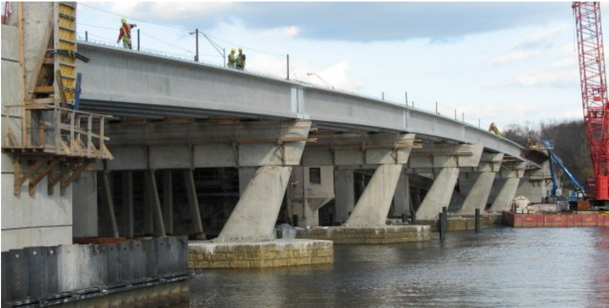
Fig. 21. Piers 1EB through 5EB have been completed and bulb tee girders erected.
