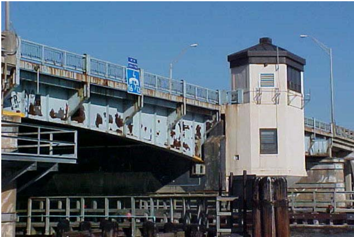
Fig. 1. Existing bridge bascule span.
