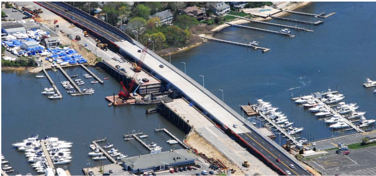
Fig. 5. Traffic has been shifted onto the newly completed eastbound half of the bridge and the existing bridge is being demolished.
