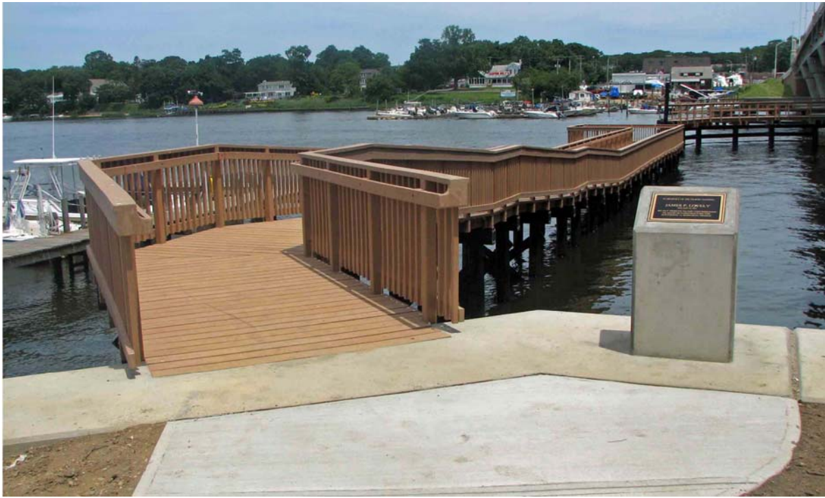
Fig. 4. Public fishing pier constructed of FRPL and FRPP.
