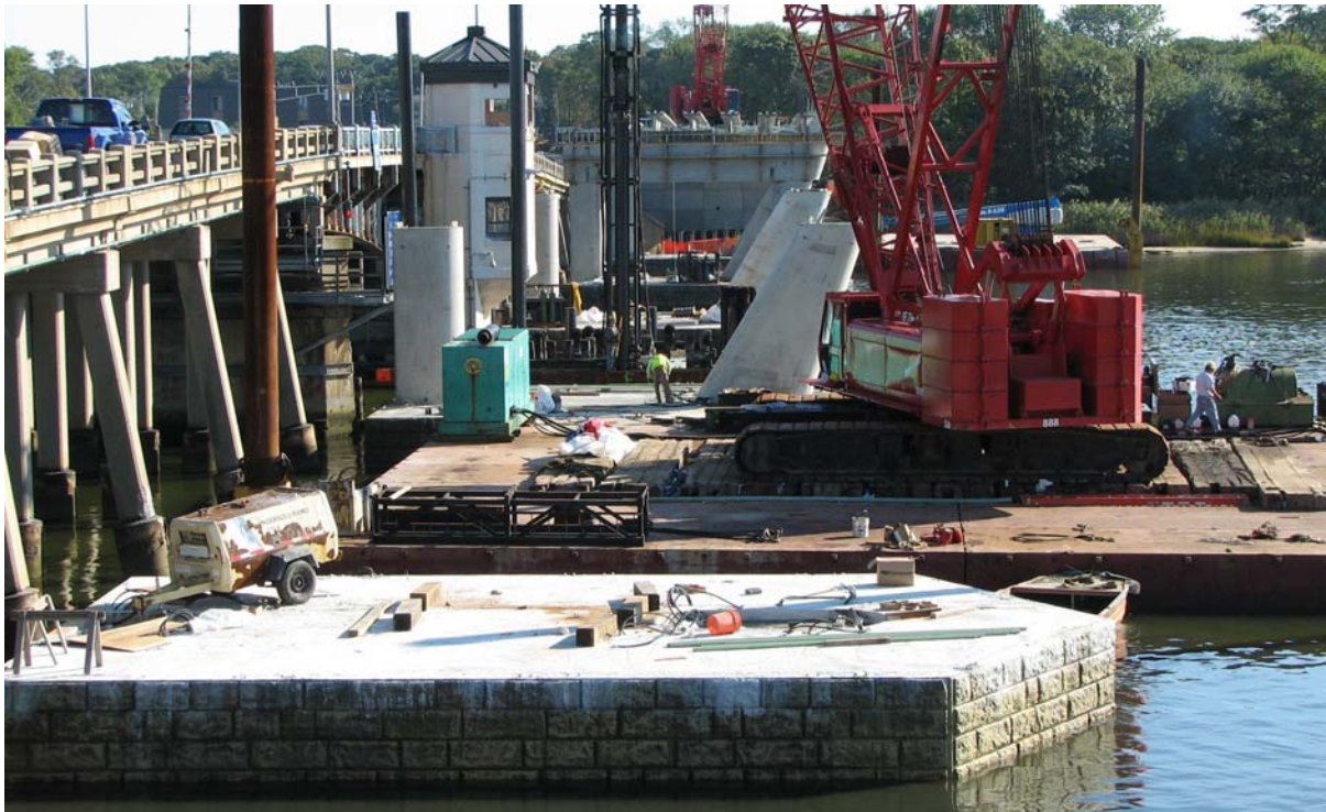
Fig. 17. Crews work on multiple piers at the same time. Piers are shown in various stages of completion.
