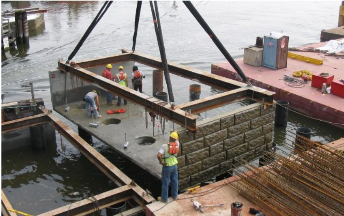
Fig. 12. Precast cofferdam section being hoisted into place.
