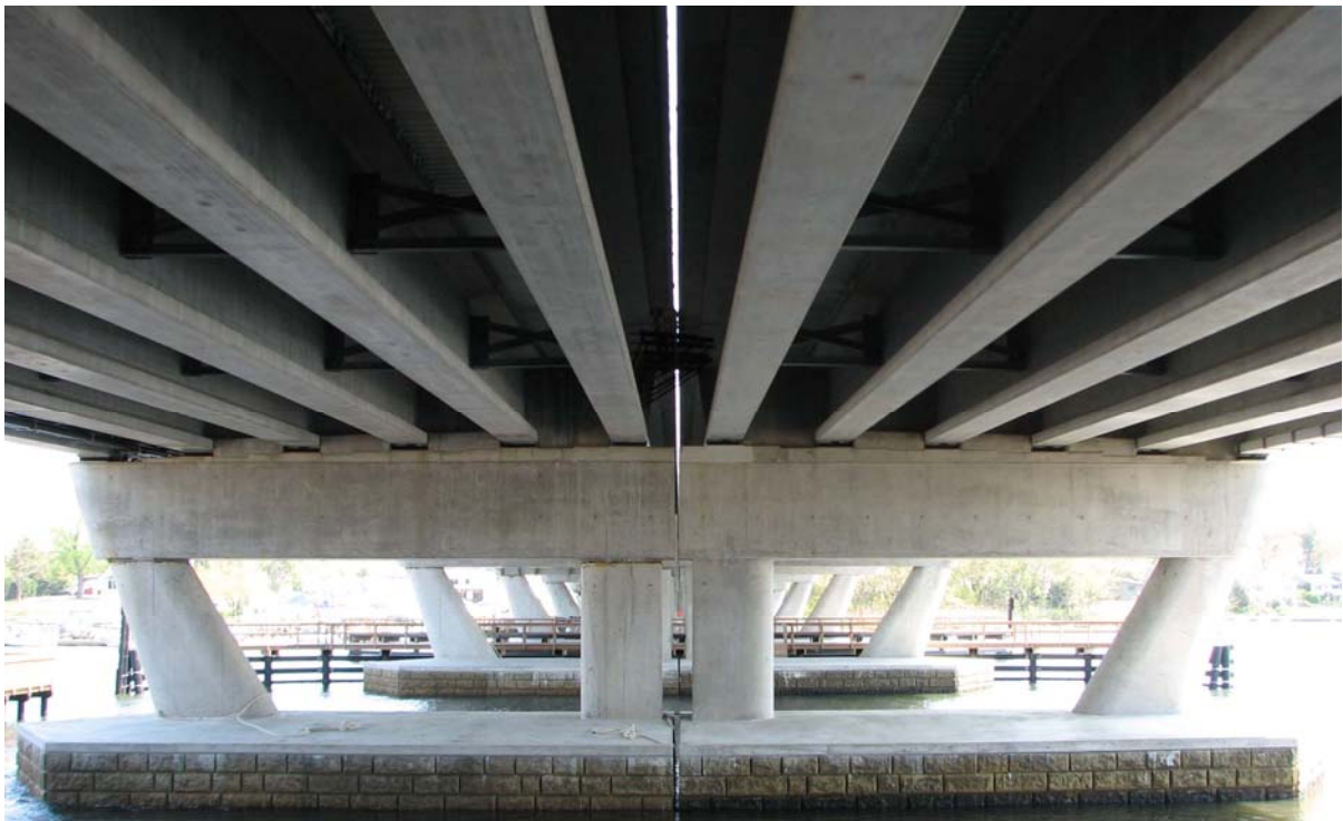
Fig. 16. All piers have been completed and the PCEF Bulb Tee girders have been erected.
