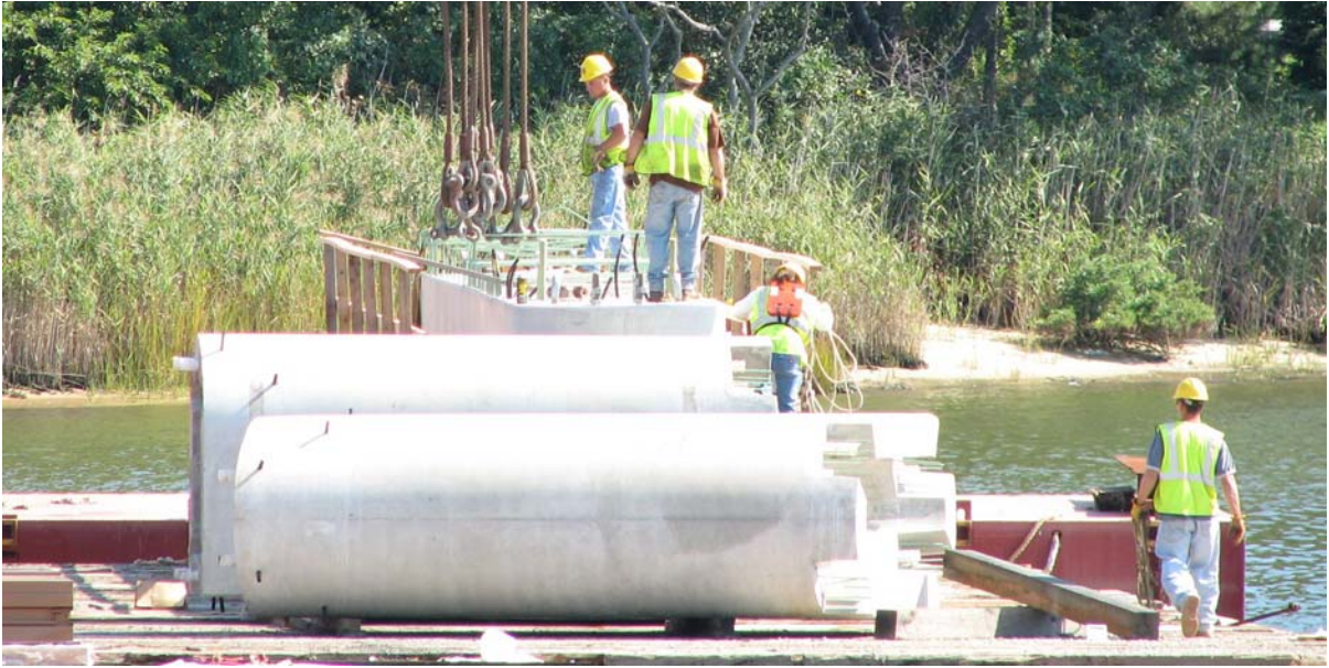
Fig. 14. Precast pier columns and a cap beam being prepared for erection.
