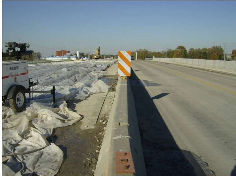
Figure 4 Phased construction of superstructure.
