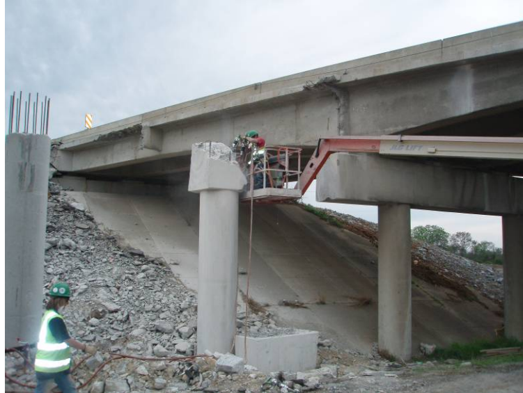
Figure 3 Removal of a portion of existing superstructure and bent cap.
