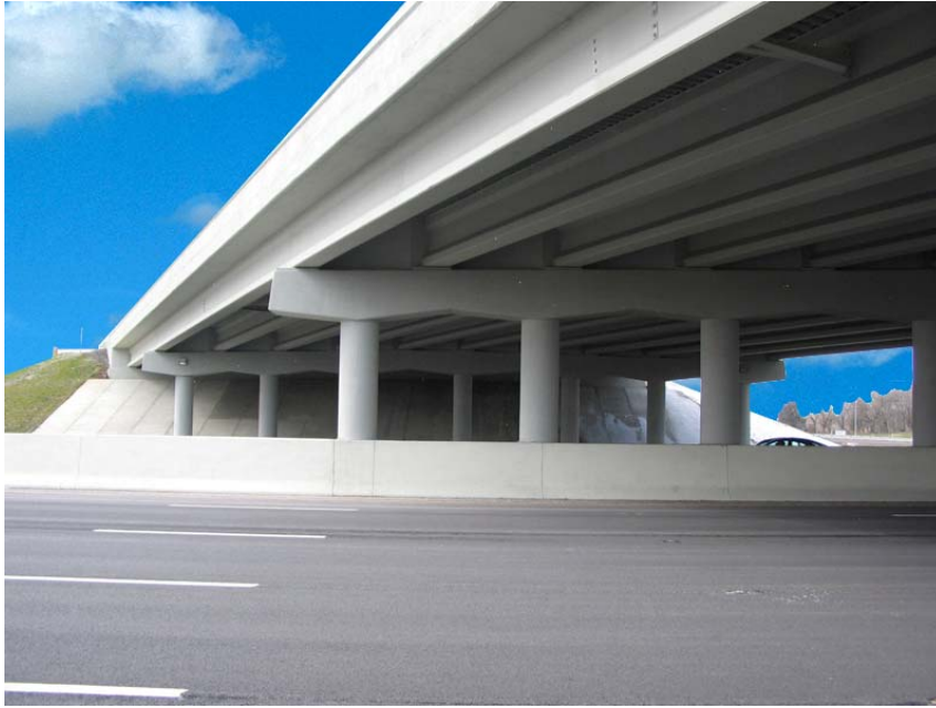
Figure 5 Bridge after widening and rehabilitation.
