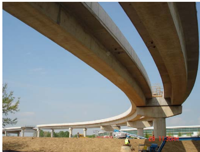
Figure 4 – Cast-in-place Girders
