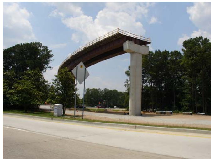
Figure 5 – Steel “Tub” Girders
