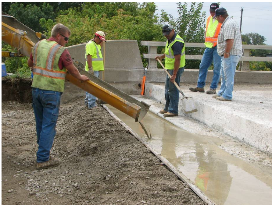
Figure 19. Backfilling the notch area with flowable mortar
