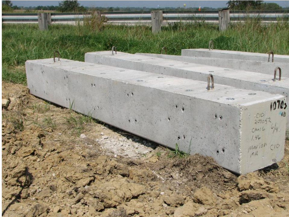
Figure 10. Precast units at the bridge site
