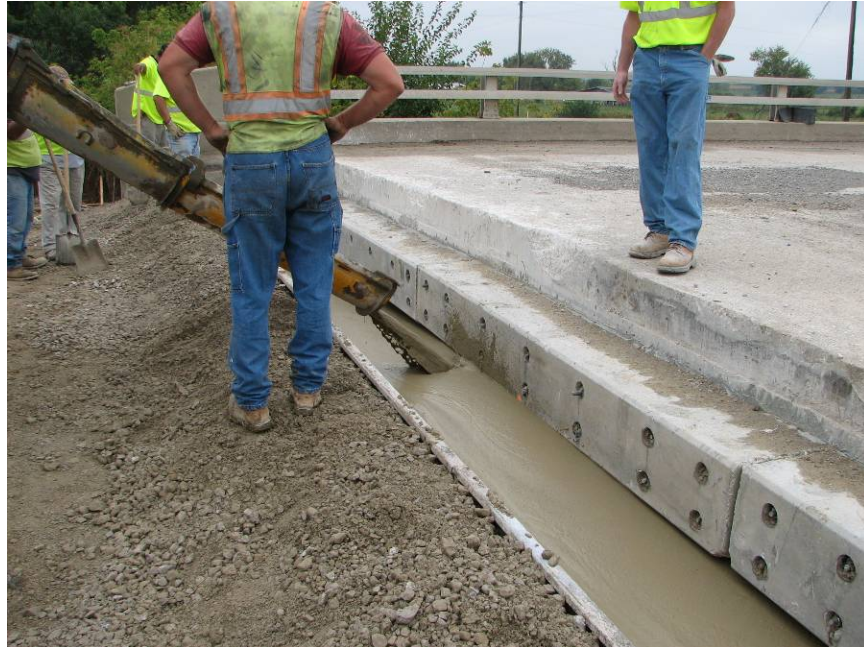
Figure 18. Backfilling the notch area with flowable mortar
