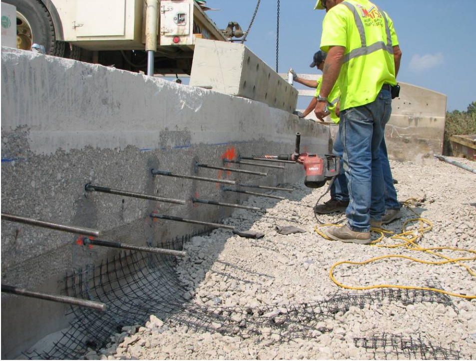
Figure 12. Drilling and installation of dowels
