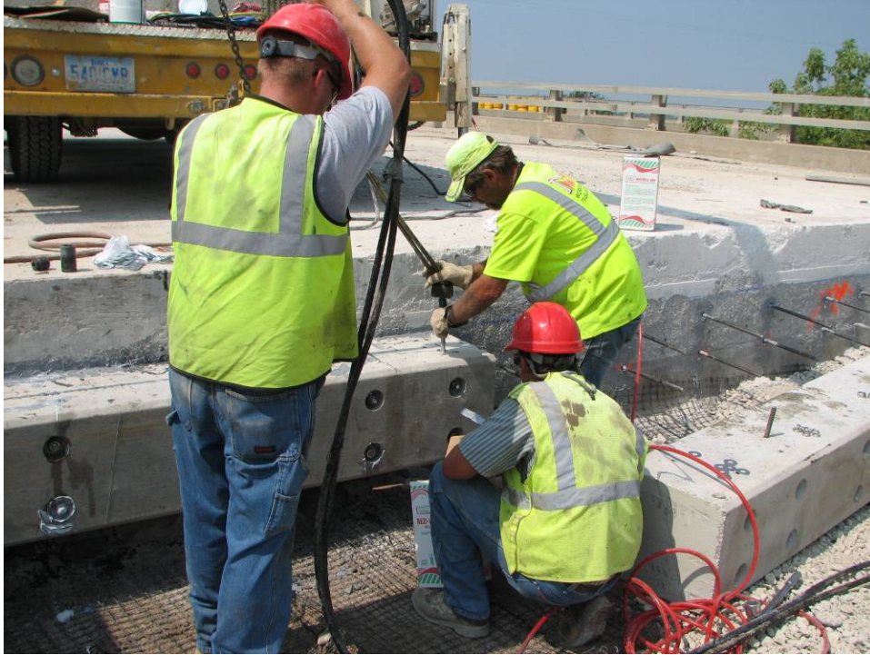
Figure 16. Grouting dowel ducts in precast units
