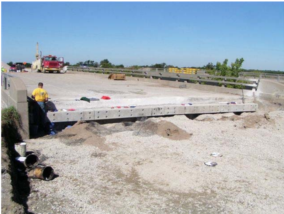
Figure 17. Final Grouting dowel ducts in precast units
