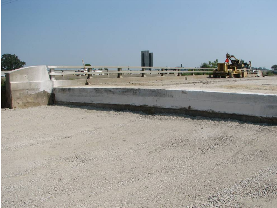
Figure 11. Existing abutment paving support removed
