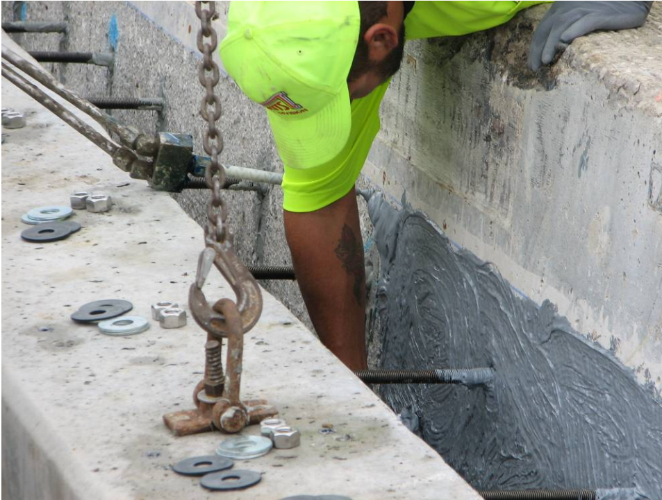
Figure 13. Applying epoxy paste to backwall
