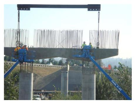
Fig. 8: Precast Bent Cap under Construction in Washington State
