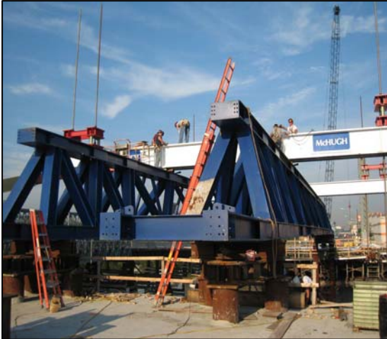
Figures 14, 15: Cross beams were used to support the lifting jack assemblies at the four corners of the bridge. Courtesy of Richard Dolan, URS Corporation
