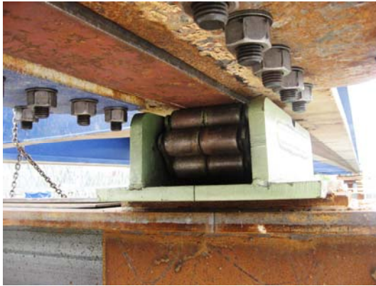
Figure 10 and 11: Roller Used to Launch the Truss, Timber Mats Used to Support the Load. Courtesy of M. Mateen, Infrastructure Engineering 5
