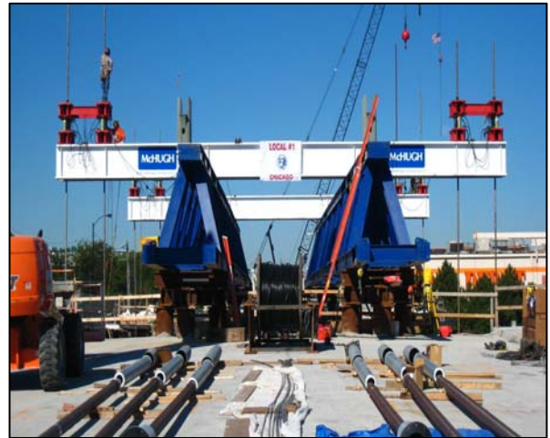
Figures 14, 15: Cross beams were used to support the lifting jack assemblies at the four corners of the bridge. Courtesy of Richard Dolan, URS Corporation
