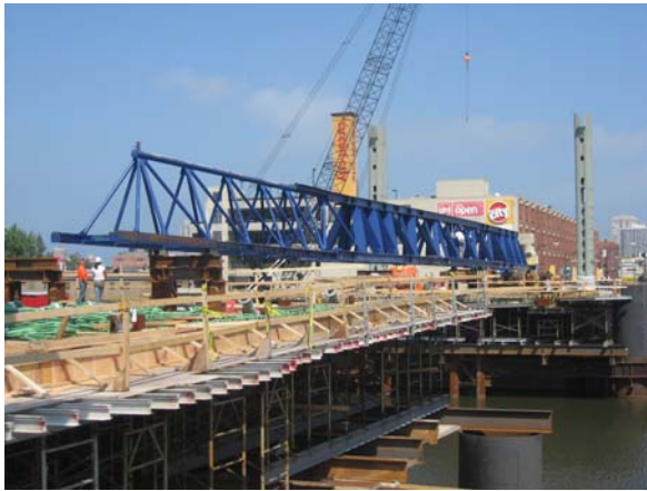
Figure 12, 13: 50 ton rollers, along with come-alongs and a grip hoist were utilized to launch the trusses across the river, Courtesy of Richard Dolan, URS Corporation 4
