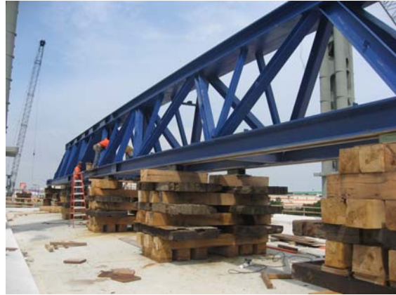
Figure 10 and 11: Roller Used to Launch the Truss, Timber Mats Used to Support the Load. Courtesy of M. Mateen, Infrastructure Engineering 5
