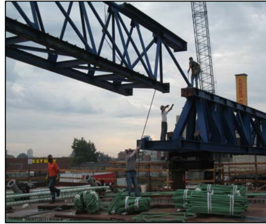
Figure 12, 13: 50 ton rollers, along with come-alongs and a grip hoist were utilized to launch the trusses across the river, Courtesy of Richard Dolan, URS Corporation 4
