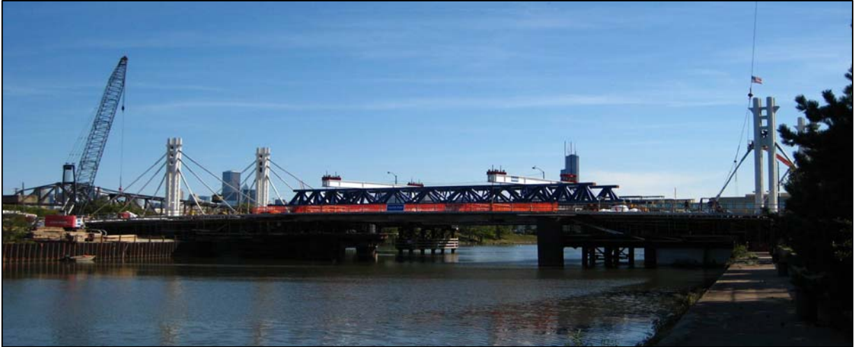
Figure 23: Center Span in Place Being Supported by the Temporary System, Courtesy of Richard Dolan, URS Corporation 4
