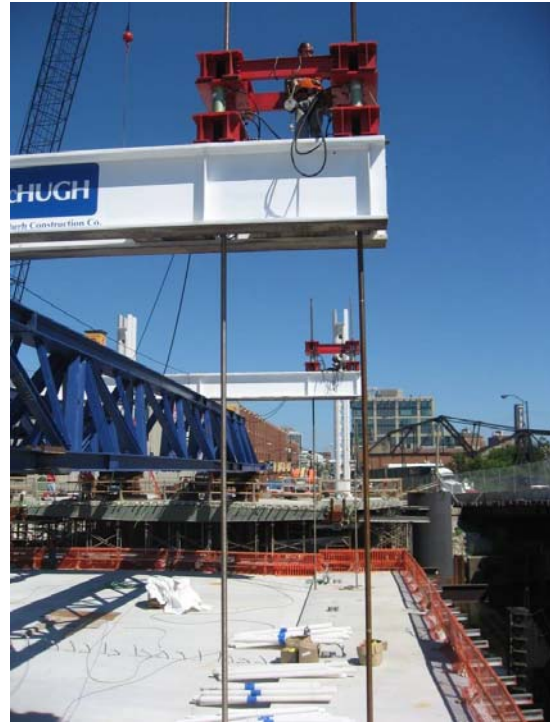
Figures 20, 21: Lifting jack Assembly from the Underside of the Span to the Top of the Temporary Structural Support Beam. Courtesy of M. Mateen, Infrastructure Engineering 5
