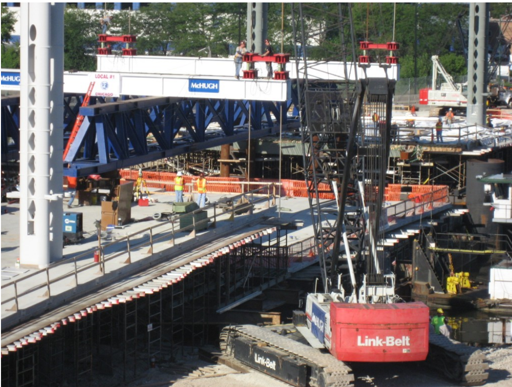
Figure 22: Center Span Lift, Courtesy of M. Mateen, Infrastructure Engineering 5
