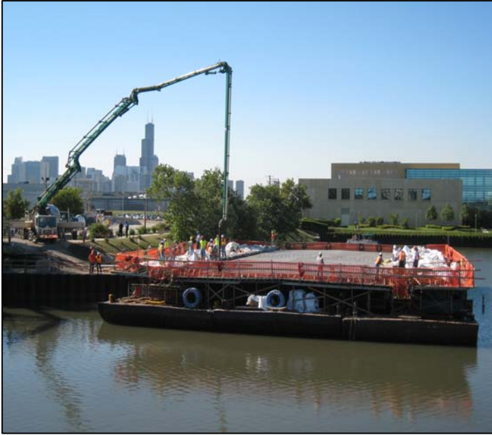
Figure 8: Composite Center Span Pour in the River, Courtesy of Richard Dolan, URS Corporation 4
