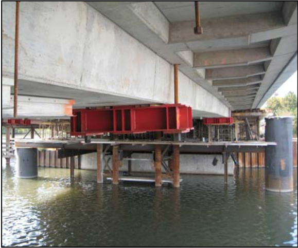
Figures 20, 21: Lifting jack Assembly from the Underside of the Span to the Top of the Temporary Structural Support Beam. Courtesy of M. Mateen, Infrastructure Engineering 5
