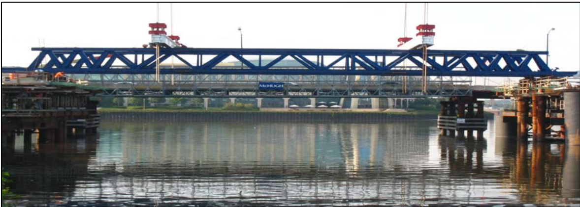
Figure 16: Center Span Lifting Assembly, Courtesy of Carlos del Val Cura, McHugh Construction 6
