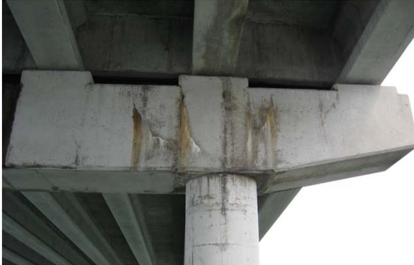
Photo 5. Typical Crack Pattern in Cantilever and Over Exterior Column
