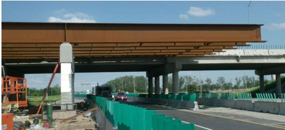
Figure 7 – Two Lanes of I-29/I-80 Each Way Maintained During Construction
