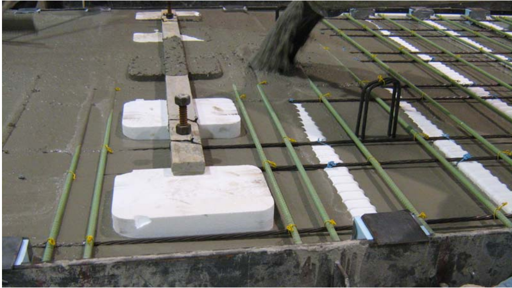
Figure 15 – Deck Panels Cast with SCC
