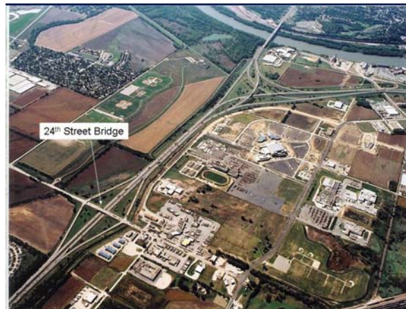
Figure 1 - Project Site Overview Looking Southwest
