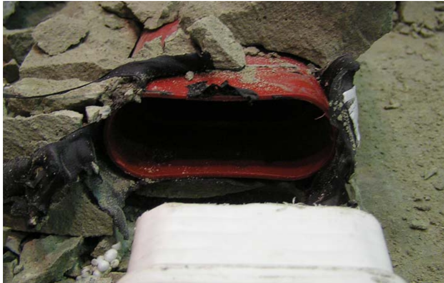
Figure 19 - Interior of a PT Duct Following Extraction
