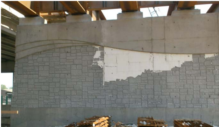
Figure 3 – Wall Pier Under Construction
