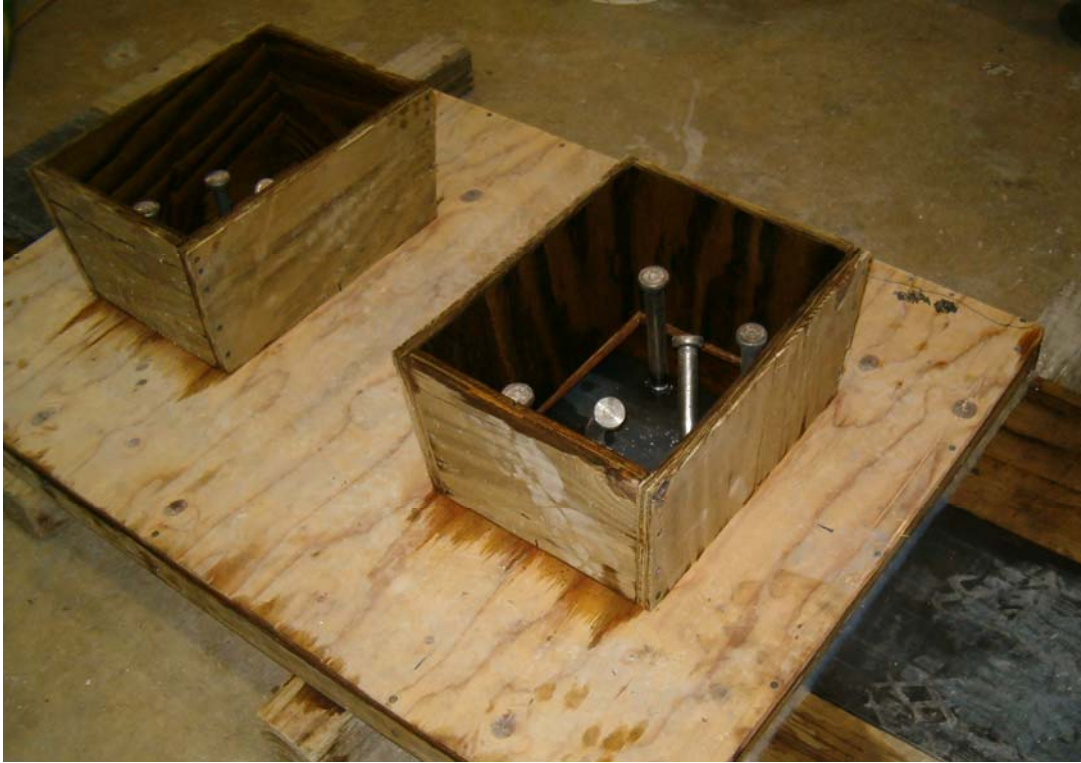
Figure 16 - Haunch and Stud Pocket Mock-up
