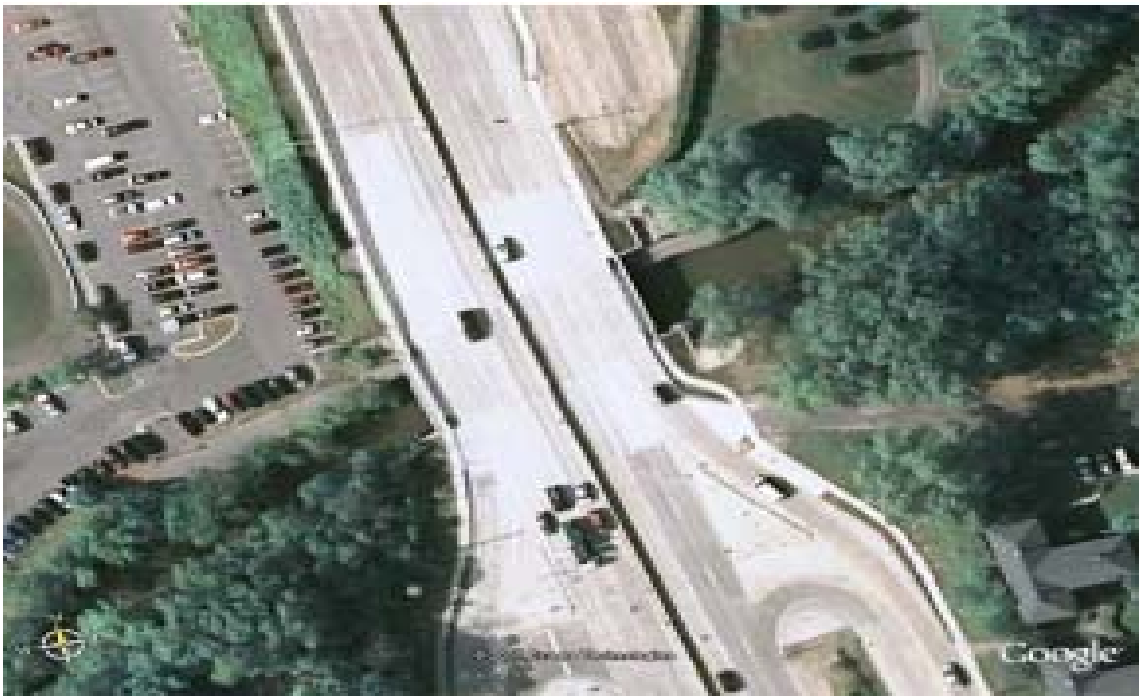
Fig. 1 – Aerial View of B01 Bridge
