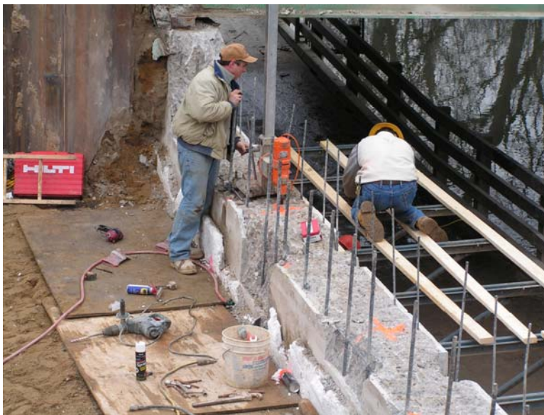
Fig. 8 - Post-Tensioning Drilling & Roof Construction
