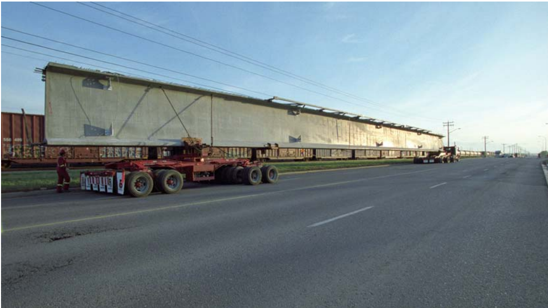
Fig. 3- A 9-ft, 3-in.-deep, 61 m (200 ft) long, 130 ton, NU I-girder, being shipped with a reinforcing steel truss attached to the top flange for additional stiffness. Courtesy of Con-Force Structures, a division of Armtec Limited Partnership, Calgary, Alberta, Canada.
