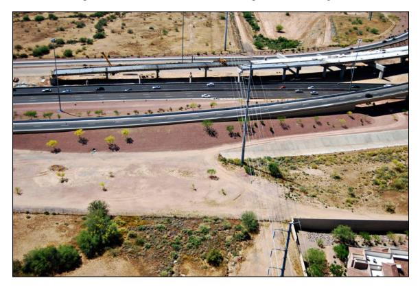
**Figure 15** – Looking south, the final abutment and four spans of the HOV SB Bridge could not be built until the detour is decommissioned and SR101L EB traffic is restored to its location under the completed portions of the HOV Bridges.
