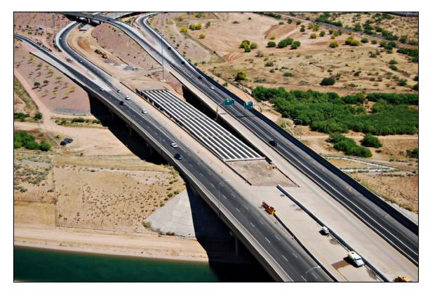
**Figure 03** – Just beyond the north levee of the CAP Canal, one 472' bridge carries SR51 HOV (SB & NB) over the Low Flow Channel of the Reach 11 Basin. At left, Ramps ES & WS merge into SR51 SB; at right NB SR51 diverges into Ramps NW & NE.
