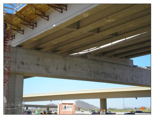
Figure 11 – Looking west, straddle bent Pier 10S supports only the HOV SB Bridge (right) while the HOV NB Bridge (left) hurdles over, clear by about 8".
