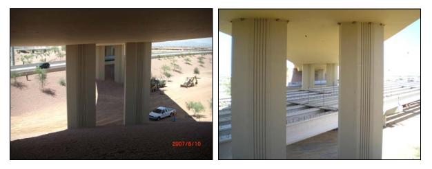
**Figure 07A and 07B** – Looking north, HOV SB and NB Bridges pass under the existing Ramp NW Bridge with limited headroom. Final Design bridge layouts move all piers and foundations out from under the shadow of the existing bridge.
