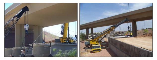
**Figures 14A and 14B** – Careful planning of pier locations proved invaluable for foundation drilling and girder setting. Shown are the two critical spans – at left looking south, is HOV SB Span 2 and, at right looking north, is HOV NB Span 1.
