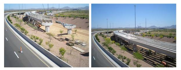
**Figures 16C and 16D** – First framing plan mobilization involves 84 girders (LT); and as deck construction has commenced, second mobilization involves 32 girders (RT).
