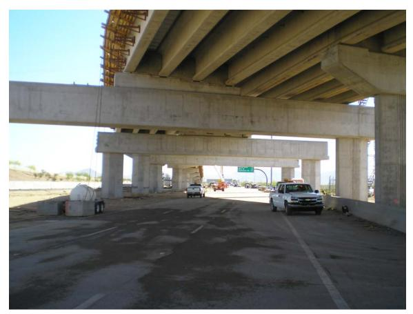
Figure 01 – First of such applications in Arizona, straddle bents support only one-of-two bridges passing over them. Pedestals constructed atop the straddle bents transfer just one superstructure load to the substructure – the other superstructure does not touch. Straddle bent Pier 10S (foreground) carries the HOV SB Bridge (LT) – but not the HOV NB Bridge (RT); Pier 10N and Pier 11N (beyond) support only the HOV NB Bridge.
