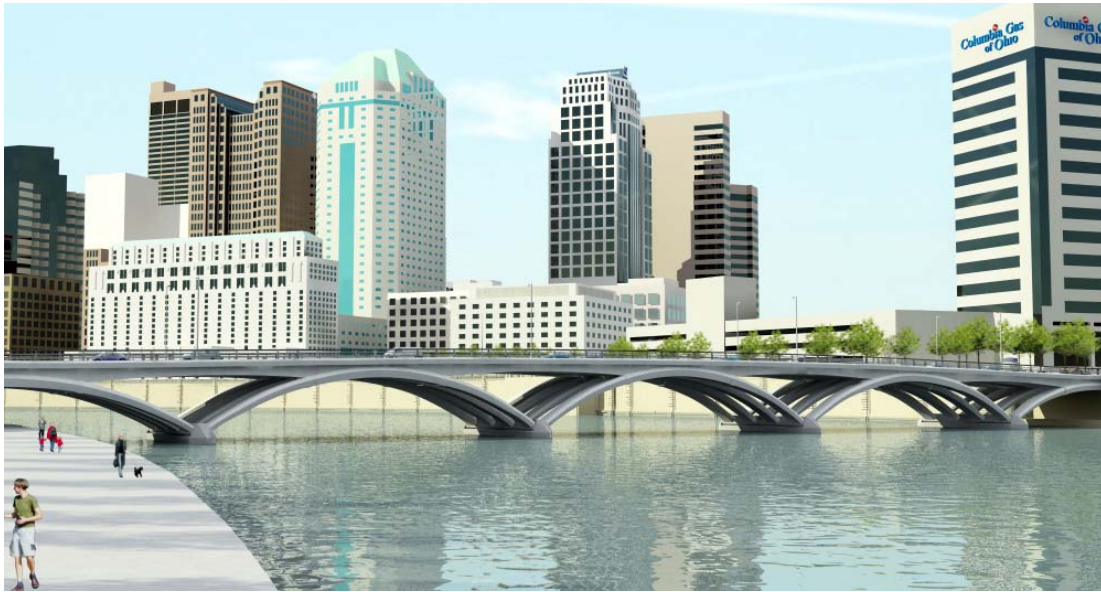
Figure 8. The new Rich Street bridge.
