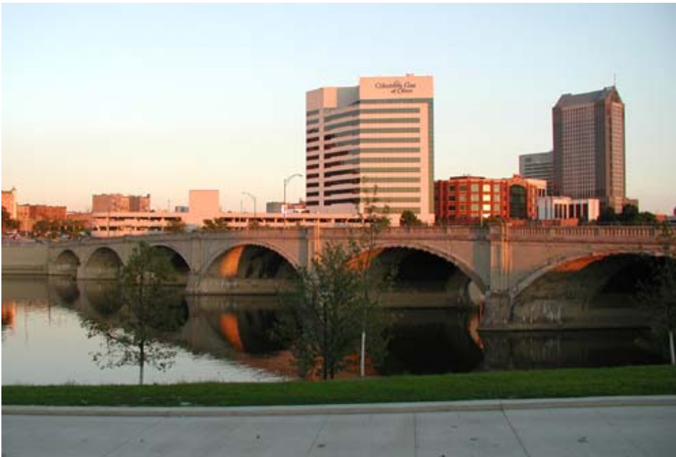
Figure 5. The existing Town Street Bridge.
