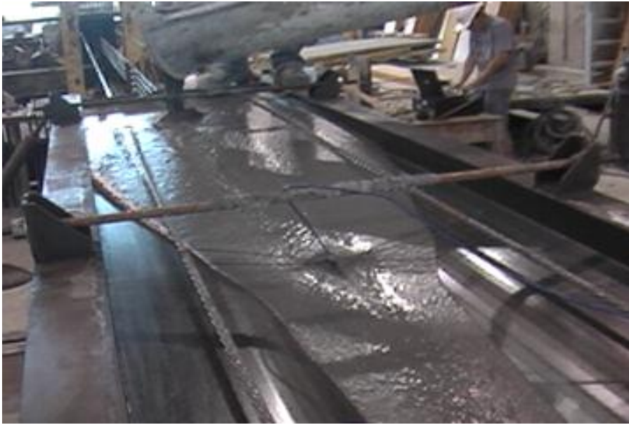
Figure 1. Casting of 110 ft. UHPC beam used on Wapello County Bridge
