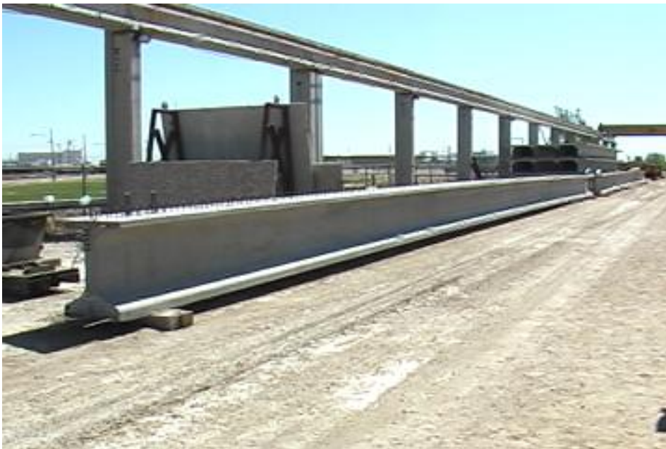
Figure 2. UHPC beams prior to shipping to bridge site in Wapello County
