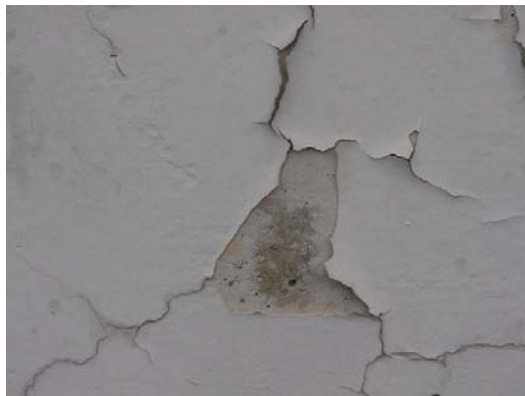
Fig. 8 Example of Bubbling and Peeling Paint
