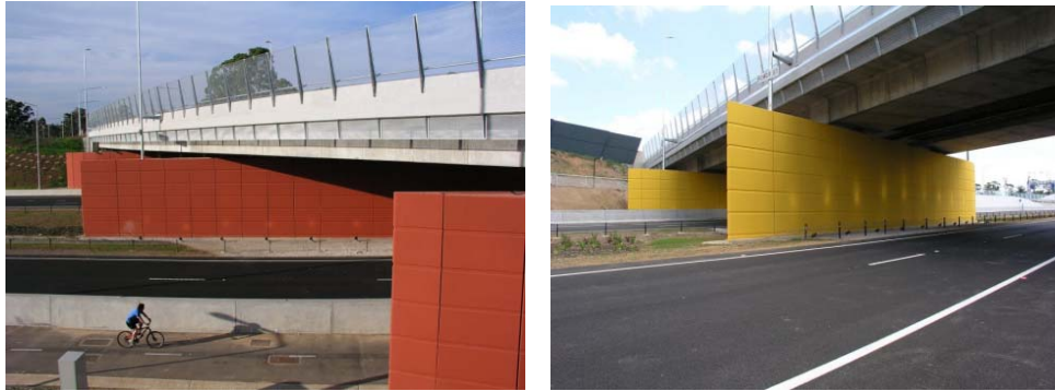
Fig. 14 Example of Color Finishes in SREP Applications
