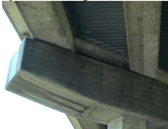
Fig. 11 Rehabilitated Pier Cap in Service
