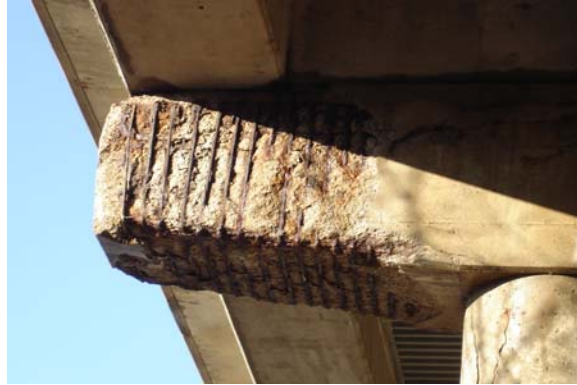
Fig. 4 Pier 7 Overhang Deterioration
