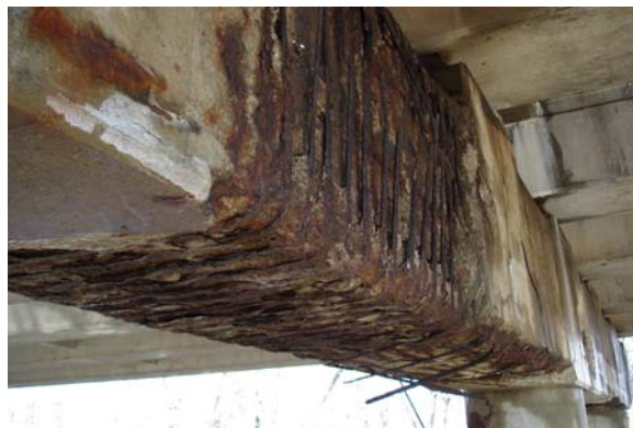
Fig. 2 Condition of Pier Caps (Pier 7 shown between columns 1 and 2)
