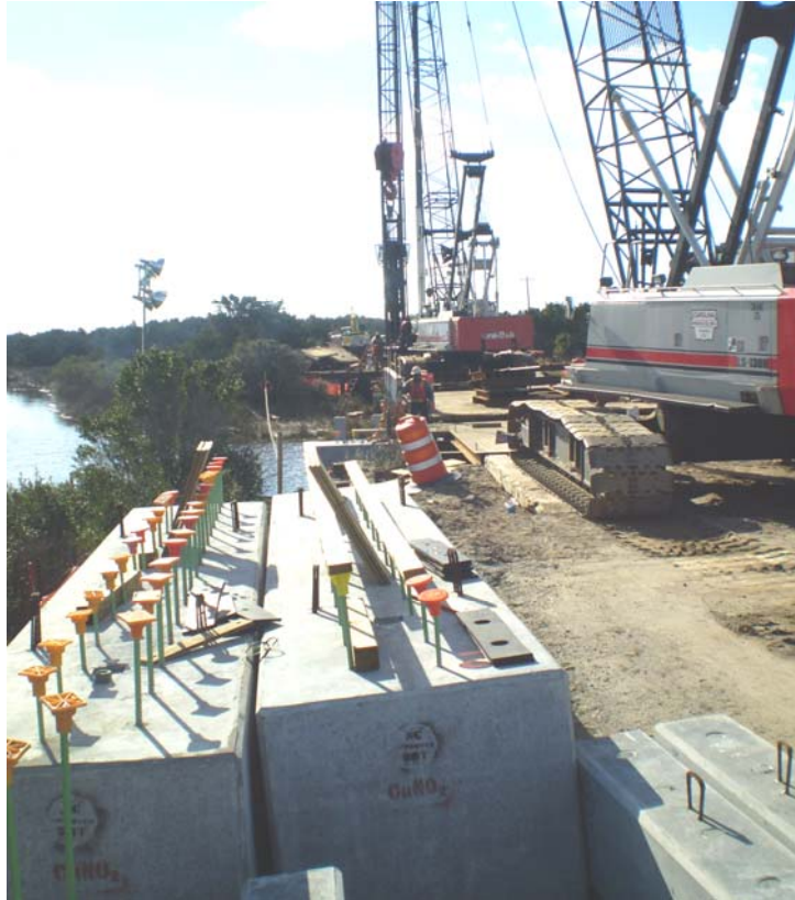
Figure 6: Substructure cap segments being placed by crane in foreground while piles are driven on the same bridge (background).
