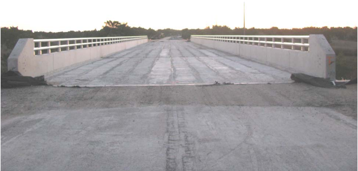
Figure 8. All precast sections in place, bridge ready for traffic.
