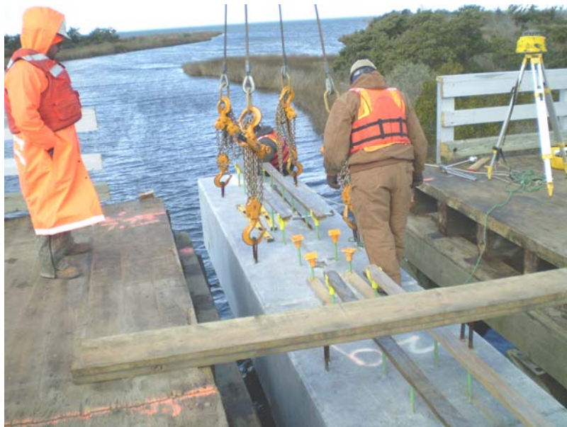
Figure 5: Precast cap segment being placed between sections of existing deck.
