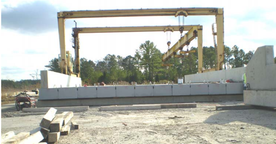
Figure 4: Mock erection at prestressing plant
