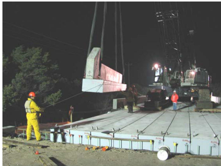
Figure 7: Field erection of precast slab and parapet.
