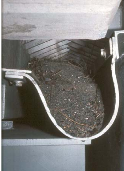
Fig. 3 Drainage Trough Filled With Debris
