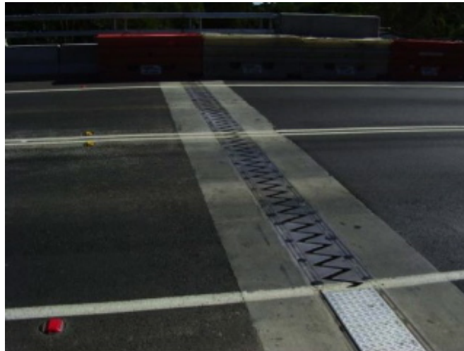
Fig. 8 SAFJ Installed on Bridge
