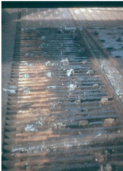
Fig. 4 Finger Plate Corrosion
