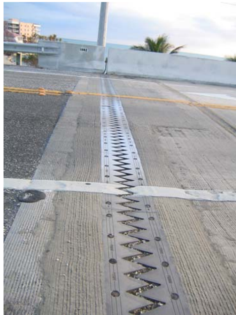
Fig. 5 Sealed Aluminum Finger Joint
