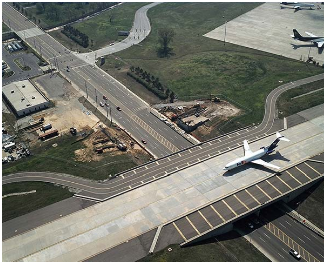
Photo 7: Bridge abutments under construction.
