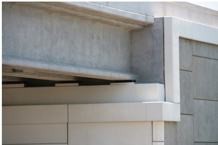
Photo 10: Close-up of integral construction technique.
