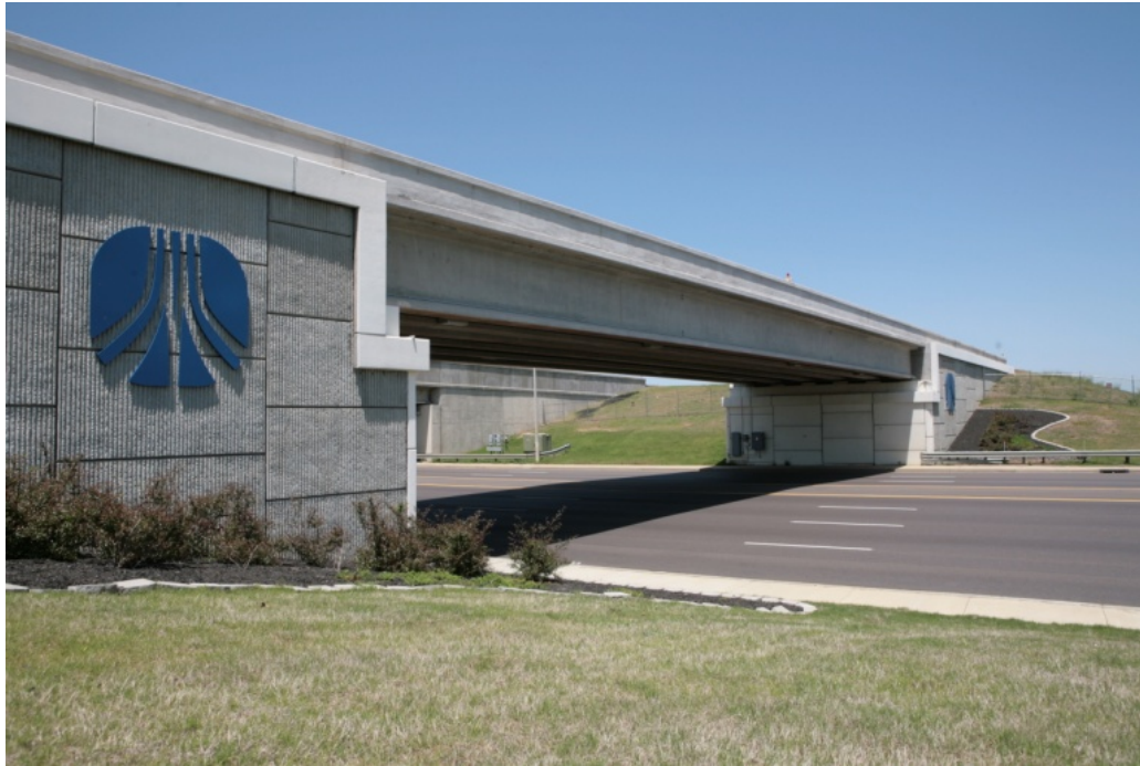
Photo 11: Winchester Service Road Bridge.
