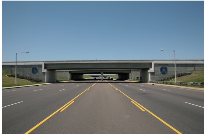
Photo 4: View of the new bridge's single span configuration.
