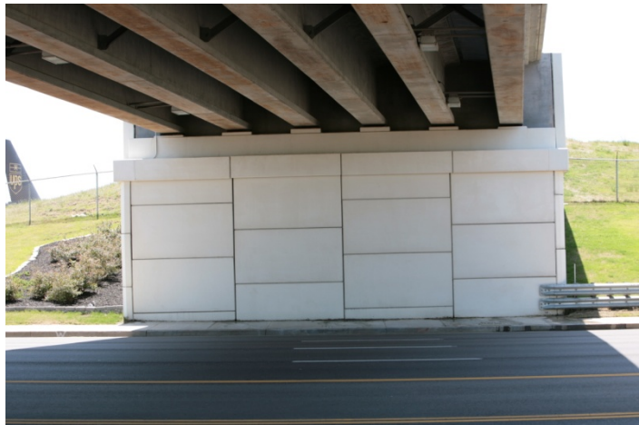
Photo 6: Girders of the new bridge.
