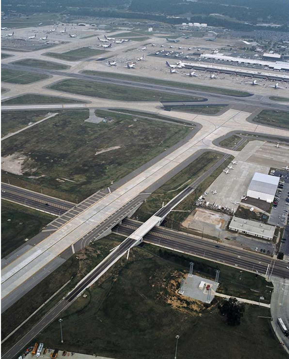
Photo 12: Winchester Service Road Bridge, aerial view.
