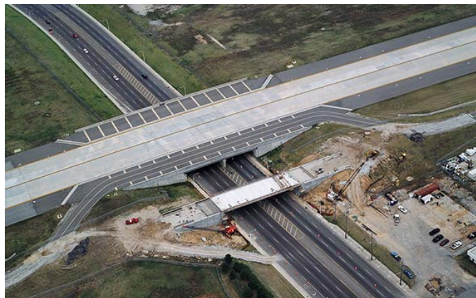
Photo 9: Construction during deck slab placement.
