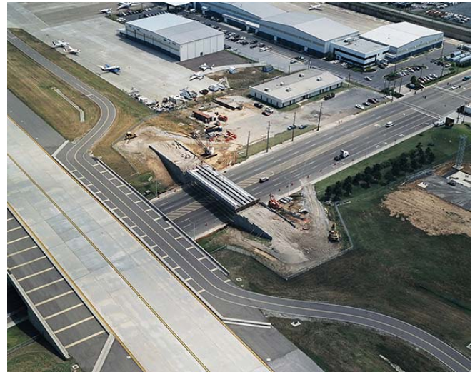
Photo 8: Construction after beams were set.
