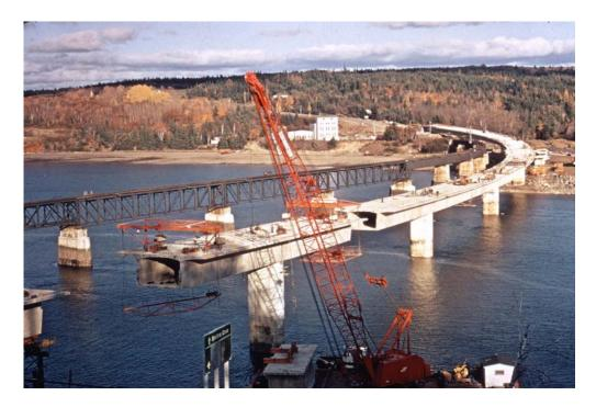
Figure 14 - Bear River Bridge (1971-1972) (first precast segmental "match-cast" bridge in North America)
