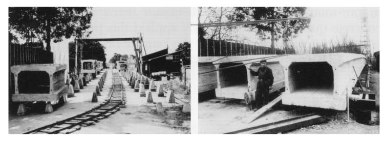
Figure 9 - Luzancy Bridge segment casting
