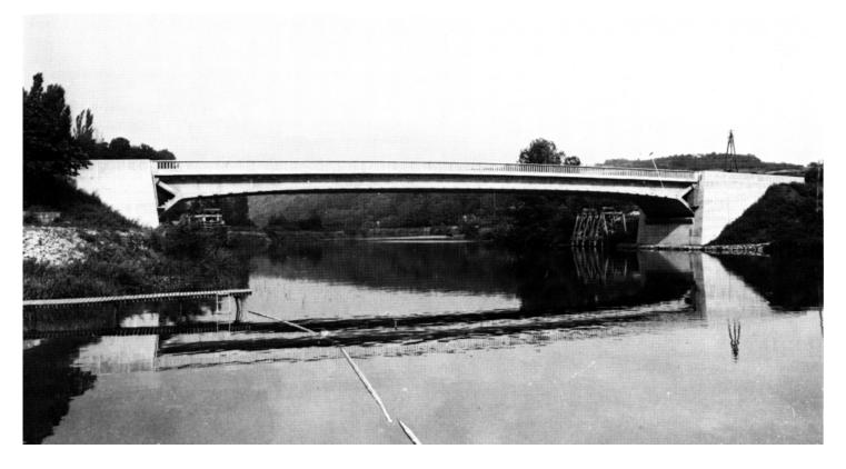
Figure 8 - Luzancy Bridge (180 ft span) (1941-1946) (first precast segmental bridge)
