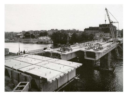
Figure 13 - Choisy-le-Roi Bridge (1962-1964) (first precast segmental "match-cast" bridge)
