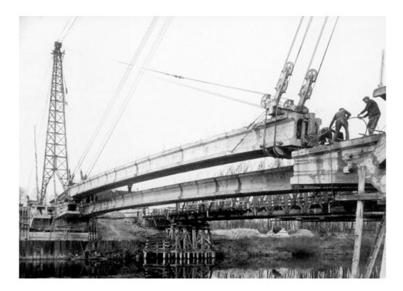
Figure 11 - Luzancy Bridge segment erection
