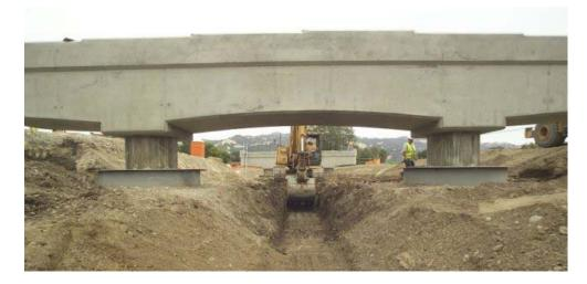
Fig. 4 Isolation of Shorter Columns at Bents 2 and 10.
