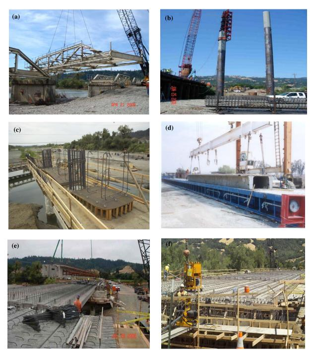
Fig. 10: Construction of the Russian River Bridge: a) Demolition of Existing Truss Bridge,
