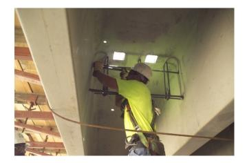
Fig. 9 Cast-in-place Intermediate Diaphragms Connecting Precast Double Tee Girders.
