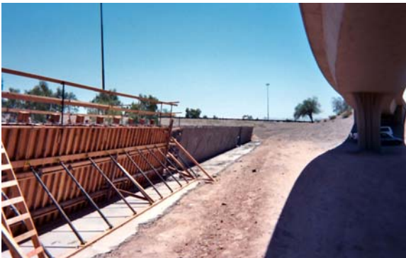
Fig. 13. Photo shows precast girders in casting yard.
