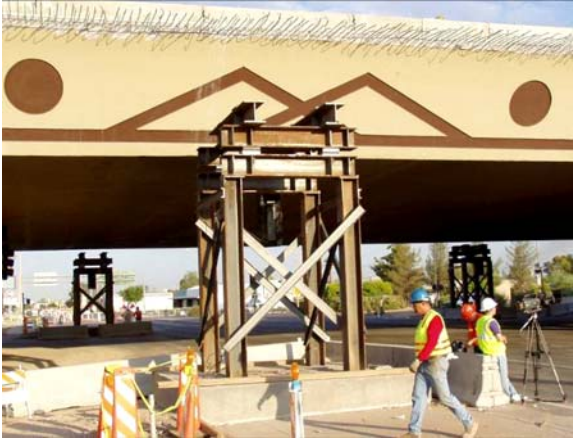
Fig. 10. This photo shows the construction of the support towers.
