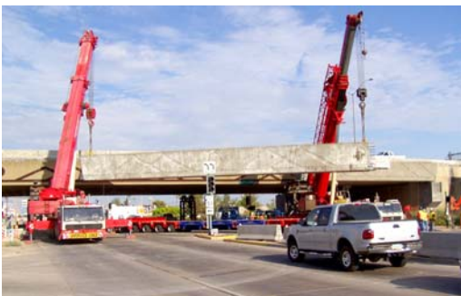
Fig. 19. Photo shows the erection of a precast girder segment.
