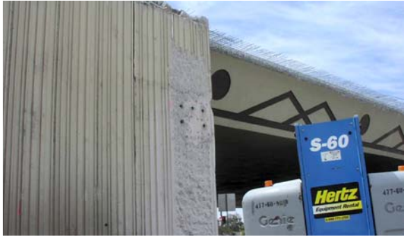
Fig. 5. This figure shows the four inch diameter by sixteen foot-long holes that were horizontal core drill in the existing abutment.
