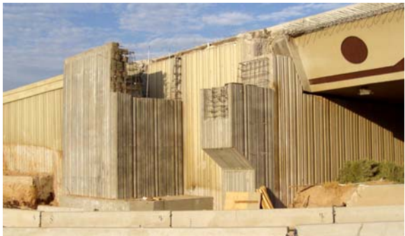
Fig. 6. This figure shows the abutment extension after it was post-tensioned to the existing abutment.
