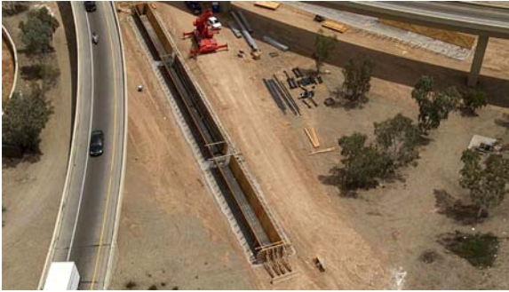
Fig. 12. Aerial photo shows precast girder casting yard.
