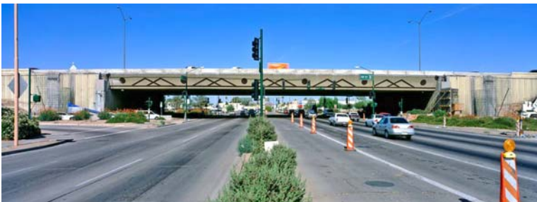
Fig. 2. This photo is of the McDowell Overpass taken at the onset of construction.
