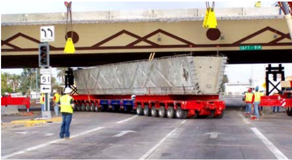
Fig. 17. Photo shows girder being transported.
