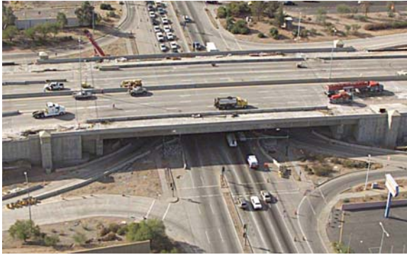
Fig. 3 This photo shows general layout concept. The main span is a simple span girder supported by abutment extensions. Short back spans were used so that the existing ramps would not need to be realigned.
