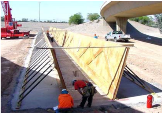
Fig. 11. Photo shows girder formwork being place on waste slab.
