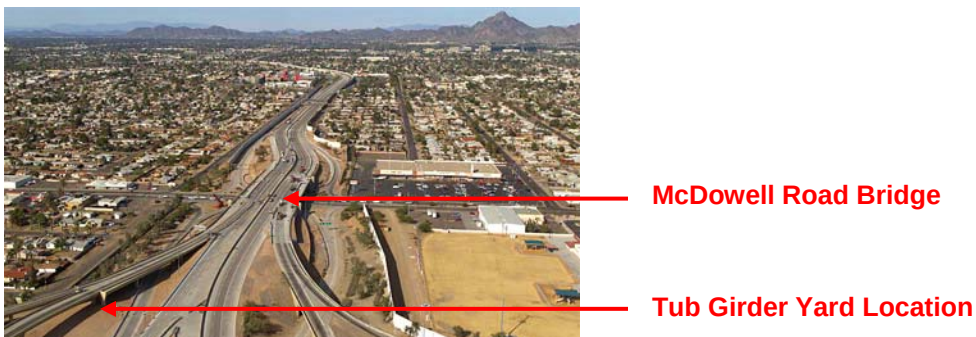
Fig. 14. This photo shows the casting yard with respect to the McDowell Overpass.
