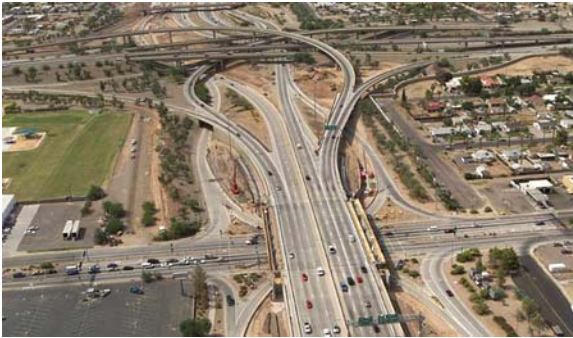
Fig. 1 This photo is looking south at the McDowell/SR51 Traffic Interchange during construction. The photo also shows I-10/SR51/SR 202L Freeway to Freeway Interchange directly south of McDowell Road.
