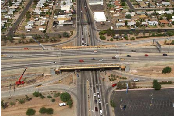
Fig. 7. This photo shows the maintenance of traffic during construction with the support towers in place.
