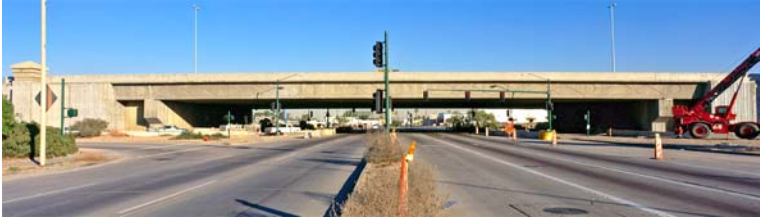
Fig. 27. Photo of completed just prior to the completion of the sound walls and painting of rustication.
