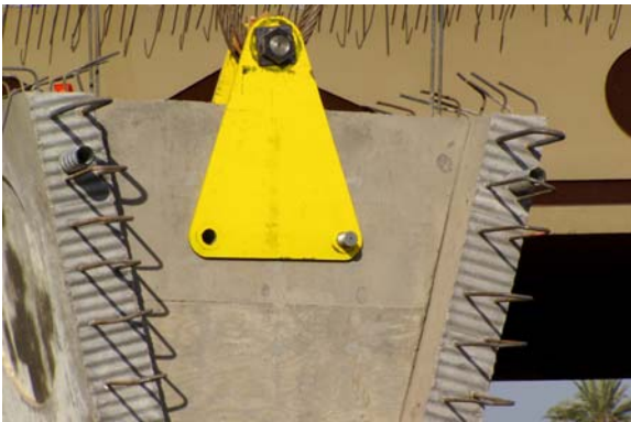
Fig. 18. Photo shows rigging begin connected to girders. Girder diaphragms were design for the girder erection loading.
