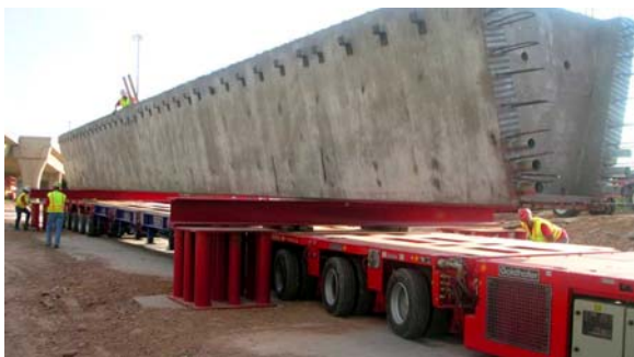
Fig 16. Photo shows girder on blocking being loaded on to transporter.
