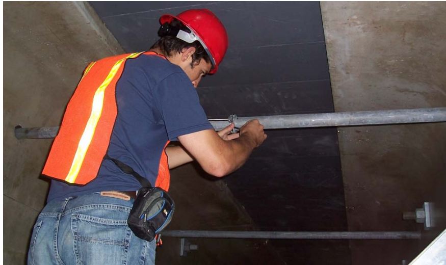
Fig. 13 Permanent instrumentation being attached to girder tie bars.
