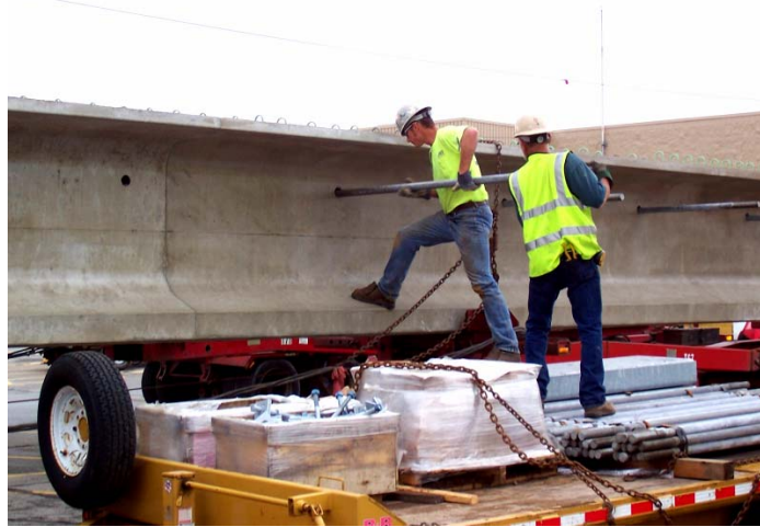
Fig. 10 Placing galvanized steel tie rods through the 54 in. bulb-Tee girders.
