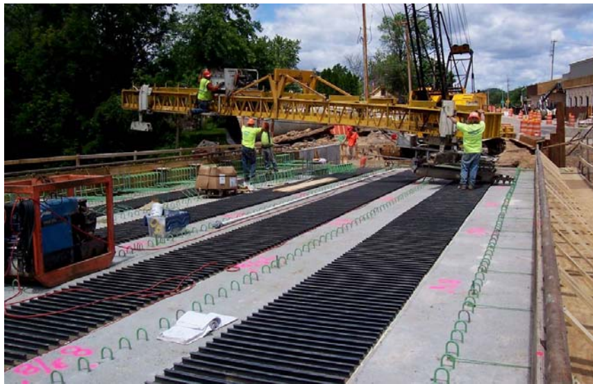
Fig. 13 Bridge superstructure before deck pour with black FRP forms.
