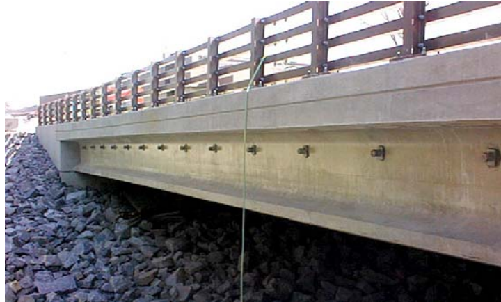
Fig. 12 Side view of bridge showing the tie rods, bearing plates and double nuts.
