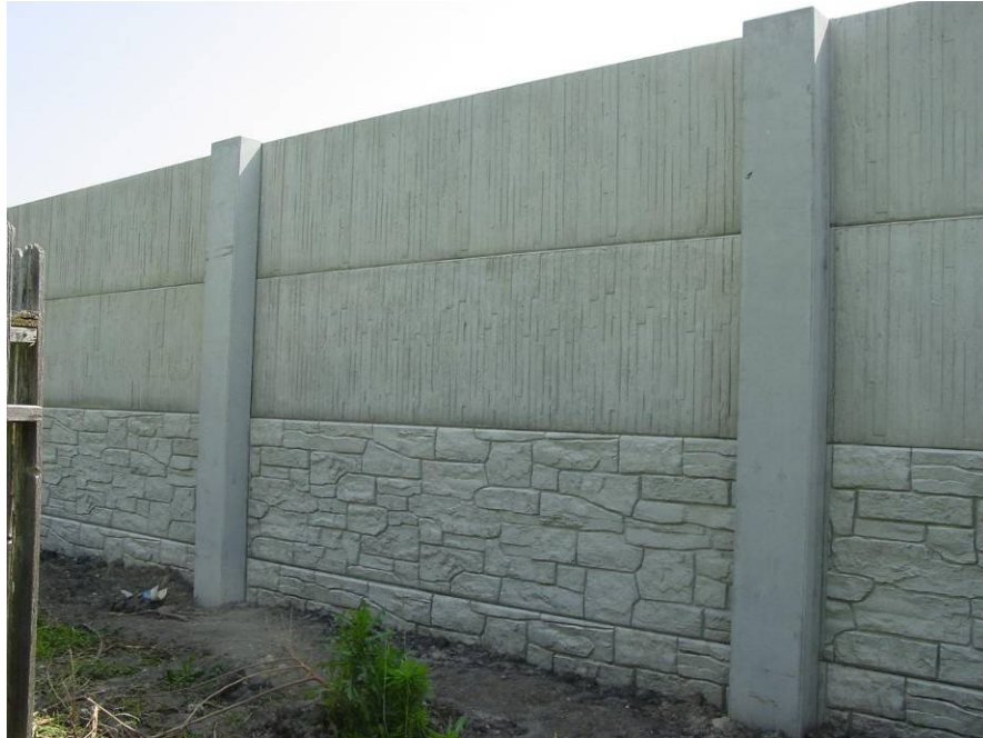
Fig.4 Sound wall residential side texture
