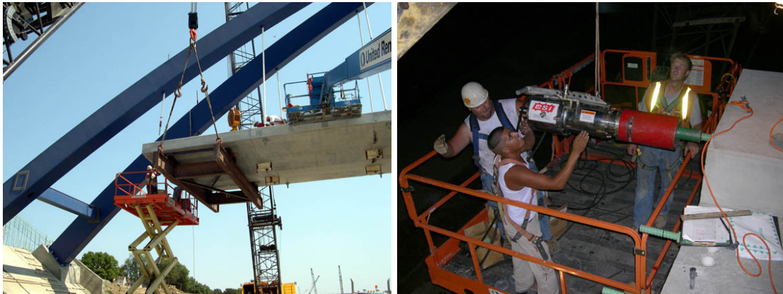
Fig. 12 Erection and post tensioning of pedestrian bridge deck panels
