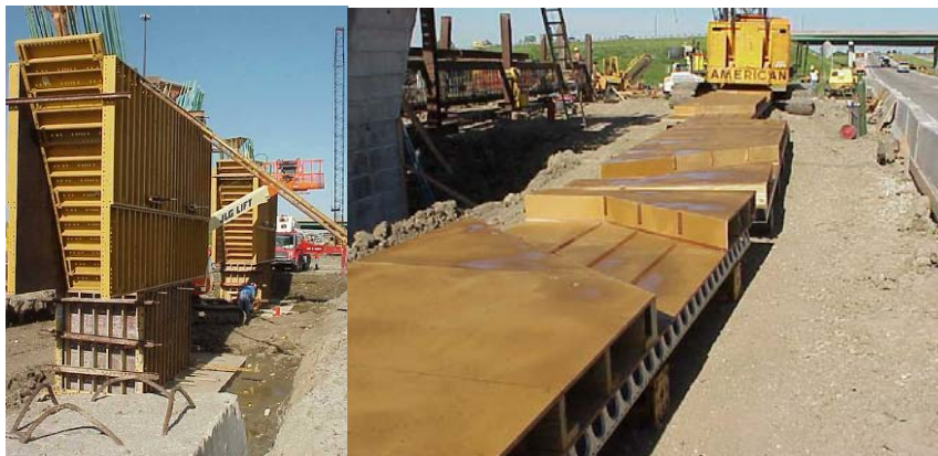
Fig. 6 Delta pier column and cap formwork
