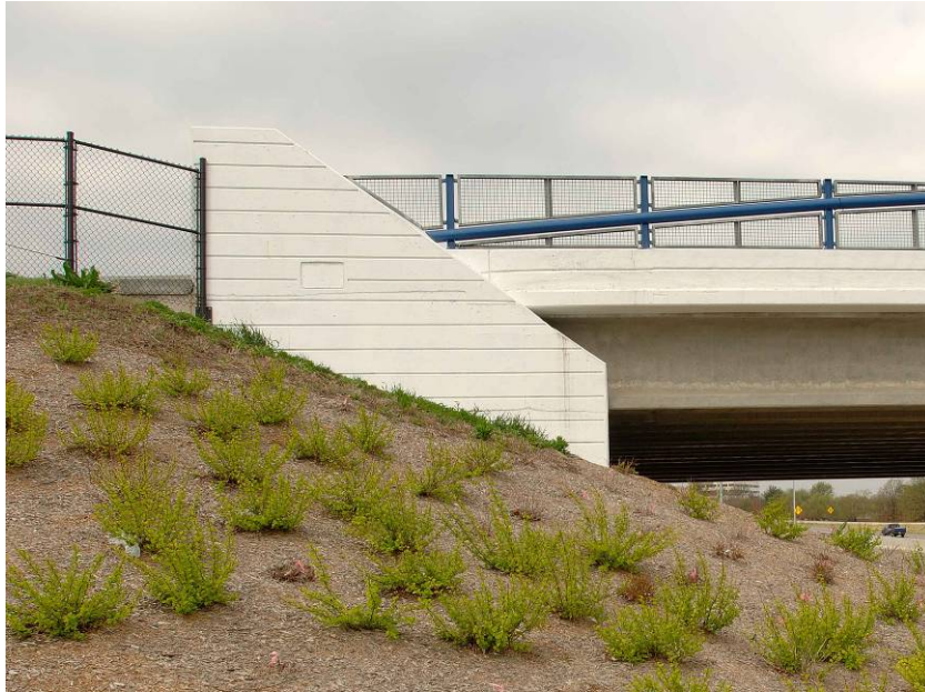
Fig. 2 Abutment end post
