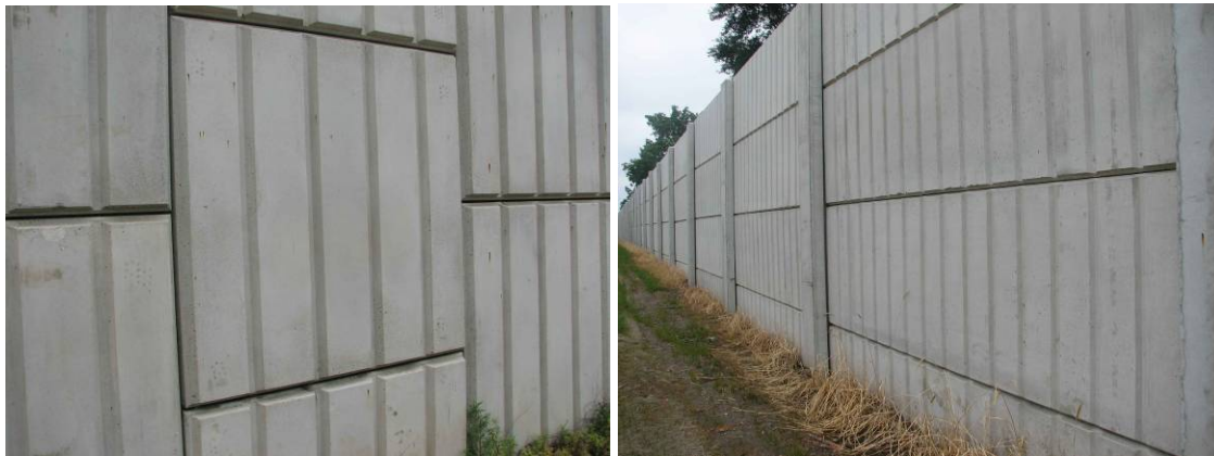
Fig. 9 MSE retaining wall and noise wall panels cast with SCC
