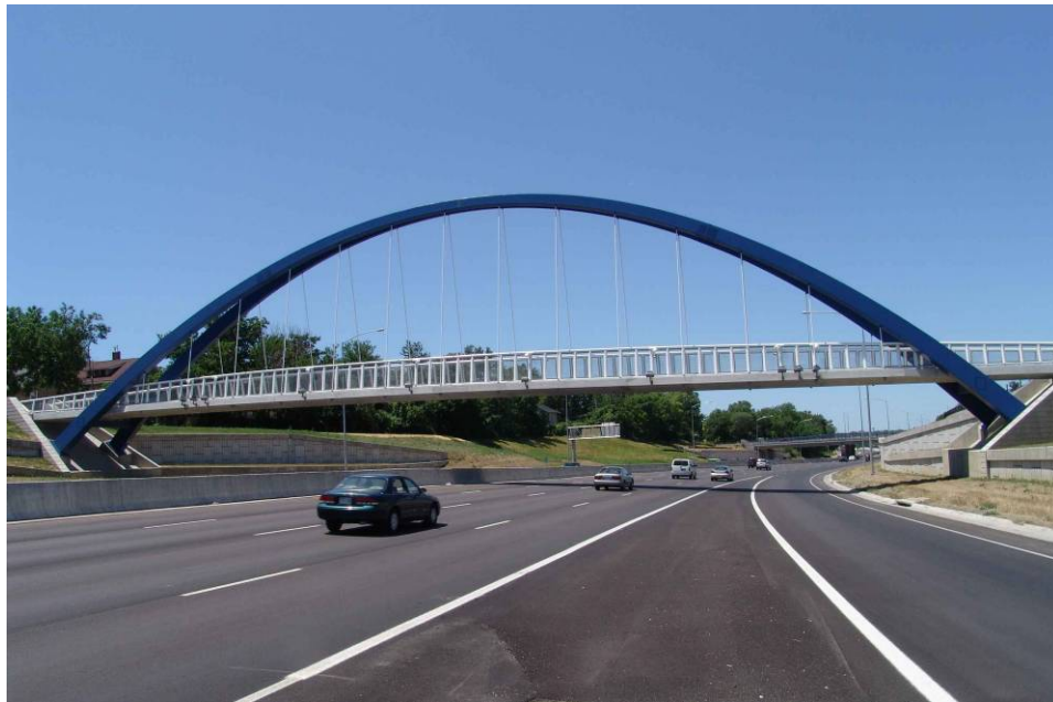
Fig. 7 Basket handle arch pedestrian bridge
