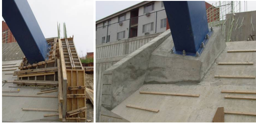
Fig. 10 SCC arch bearing pad formed (left) and result (right)
