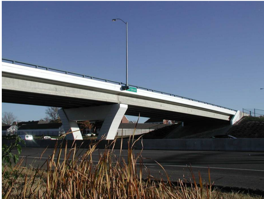
Fig. 8 Coated bridge concrete
