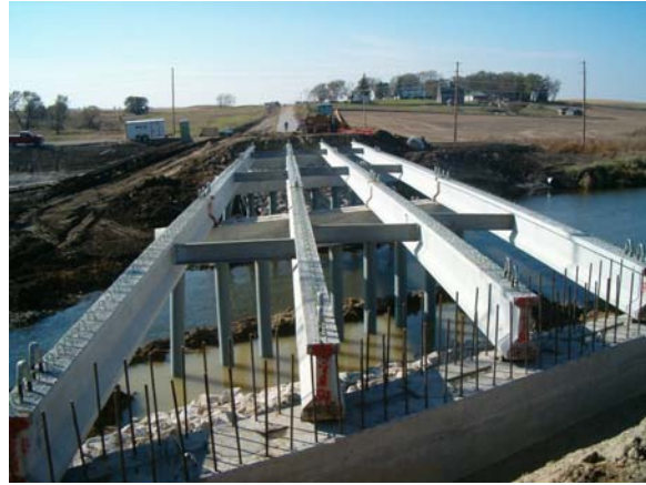
Figure 34 – PPC Beams Erected
