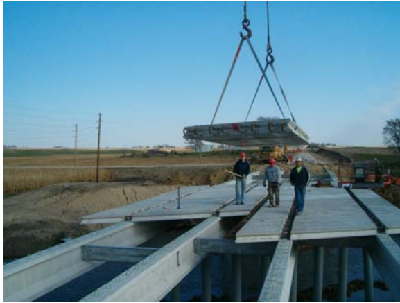
Figure 37 – Deck Panel Erection
