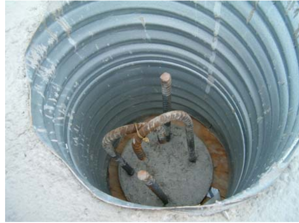
Figure 26 – Pier CMP Blockout
