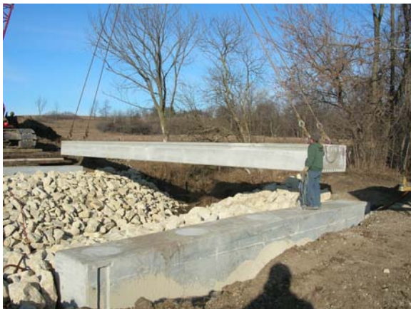
Figure 70 - Photographic timeline of typical box beam placement
