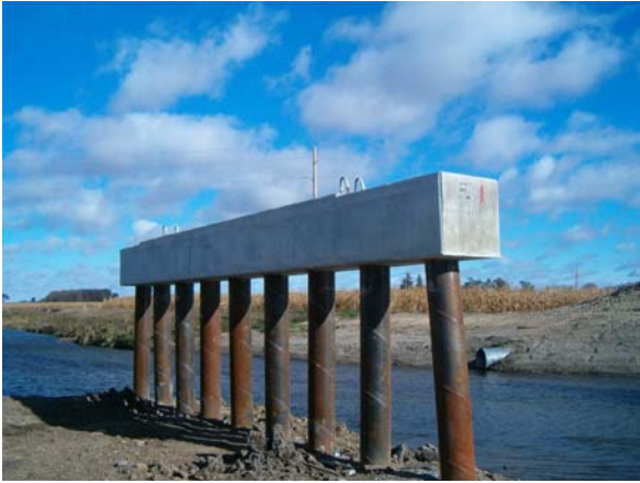
Figure 29 – West Pile Bent
