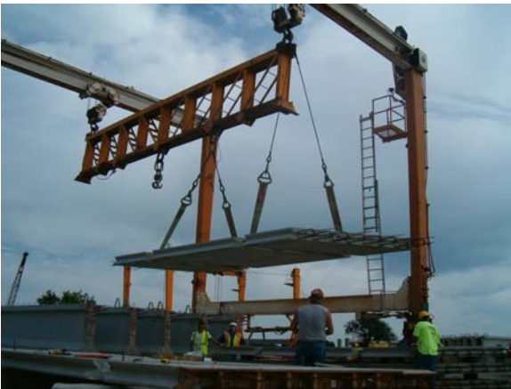
Figure 21 – Deck Panel Stockpiling
