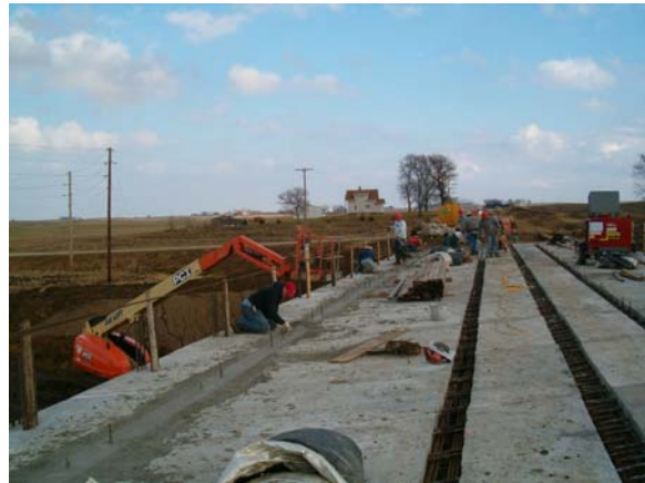
Figure 45 – Casting Long. Joints
