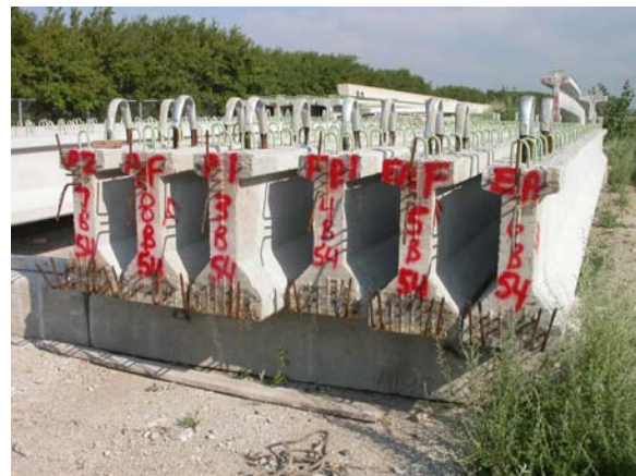
Figure 22 – PPC Beams Stockpiled
