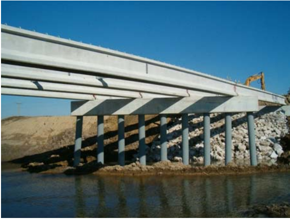
Figure 33 – PPC Beams Erected
