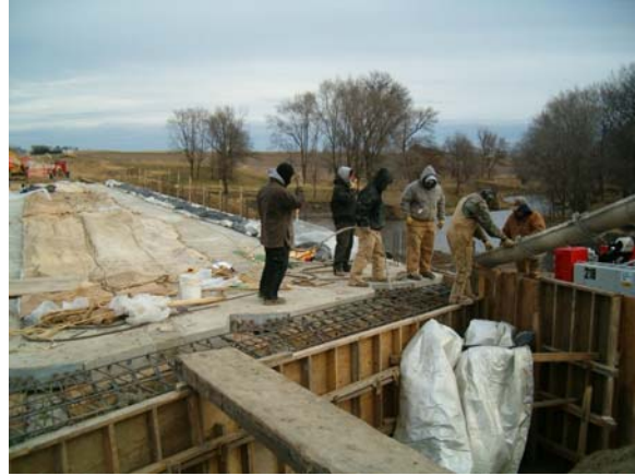
Figure 49 – CIP End Diaphragm
