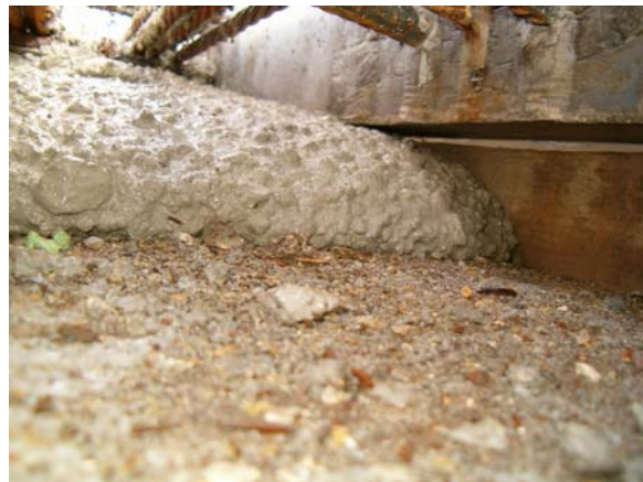
Figure 47 – Concrete Consolidation
