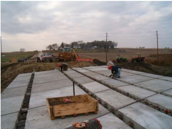
Figure 38 – Leveling Device Installation
