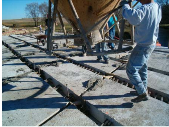
Figure 41 – Casting Transverse Joints
