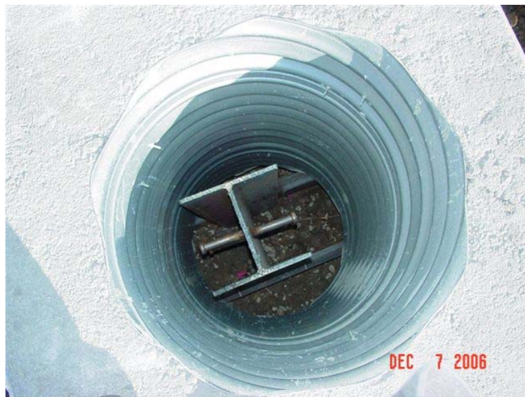
Figure 69 - Detail of the pile to abutment connection
