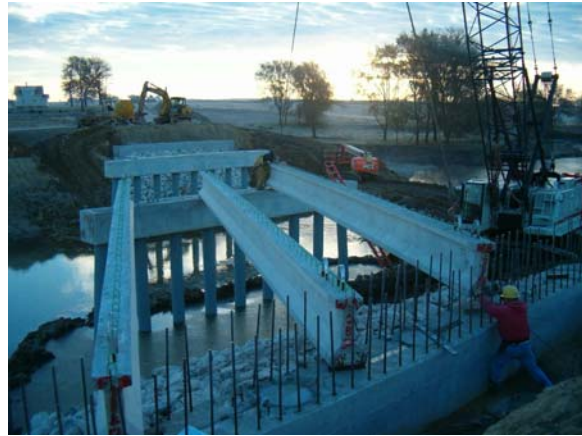
Figure 32 – PPC Beam Setting
