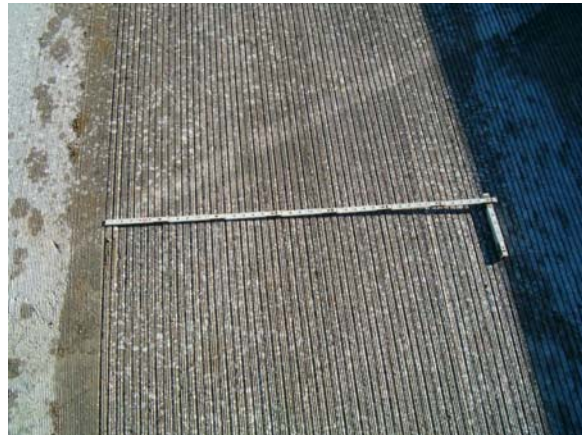
Figure 51 – Longitudinal Grooving
