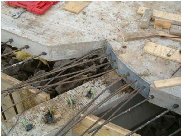
Figure 42 – PT Strand Anchorage
