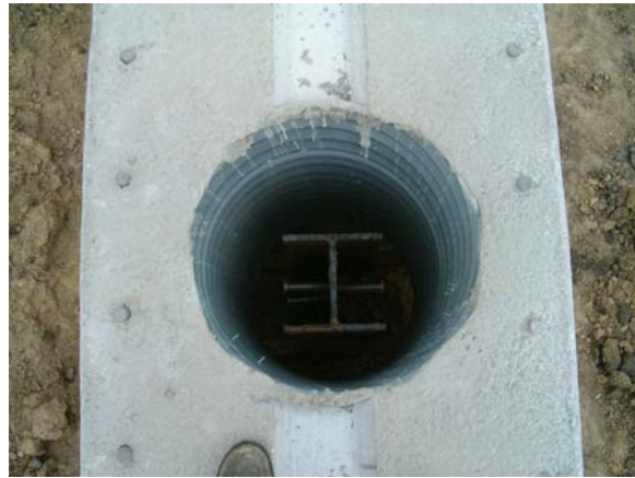
Figure 24 – Abutment CMP Blockout
