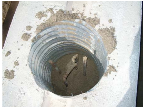
Figure 28 – Filling Pier Blockout
