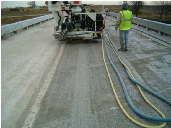
Figure 50 – Longitudinal Grooving
