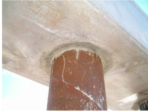
Figure 30 – Pier Cap Connection
