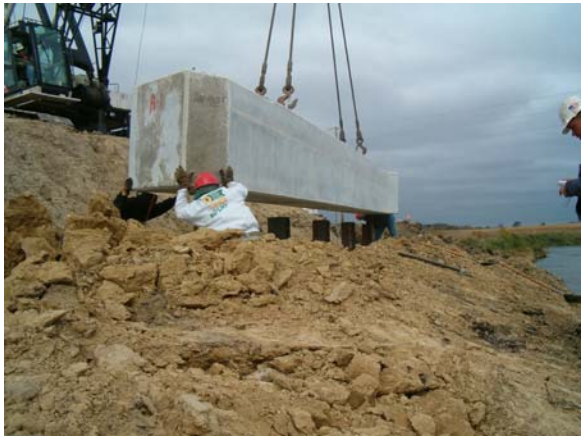
Figure 23 – Setting Precast Abutment
