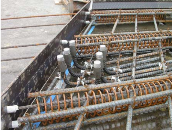
Figure 19 – Mechanical Splicers
