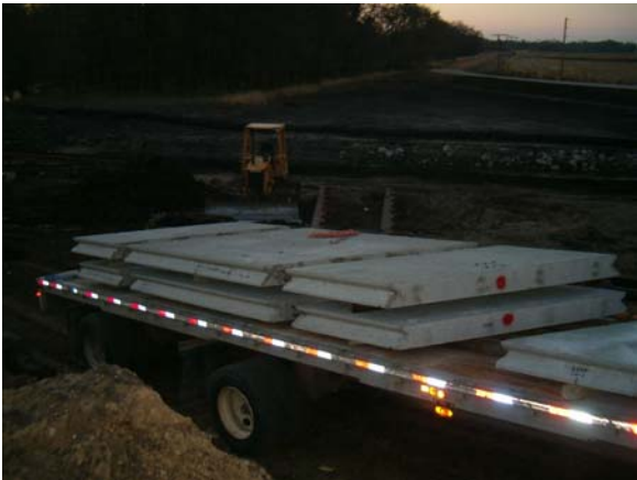
Figure 35 – Deck Panel Delivery
