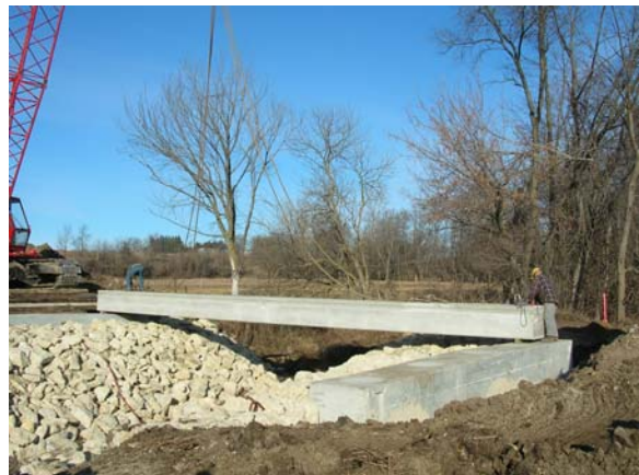
Figure 70 - Photographic timeline of typical box beam placement
