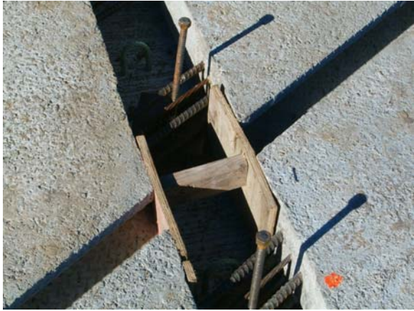
Figure 40 – Transverse Joint Form
