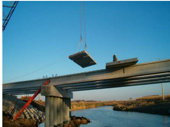
Figure 36 – Deck Panel Erection
