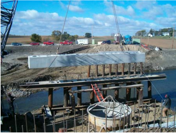
Figure 25 – Setting Precast Pier Cap
