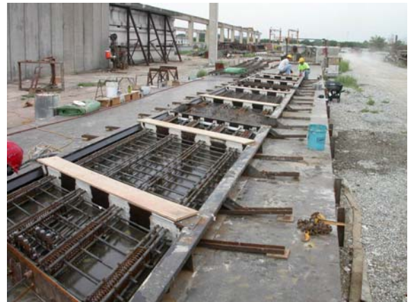
Figure 16 – Panel Form and Reinforcing
