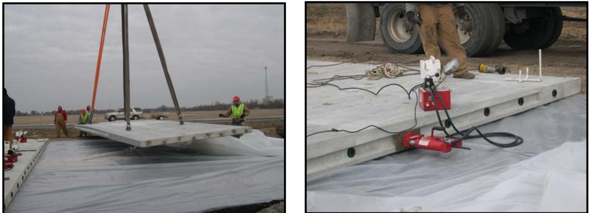
Fig. 3 Precast, post-tensioned pavement as constructed in Missouri
