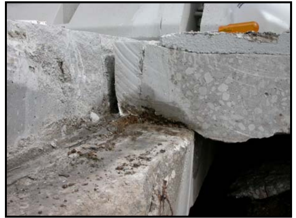
Fig. 4 Bridge approach pavement settlement and damage caused by erosion and construction errors
