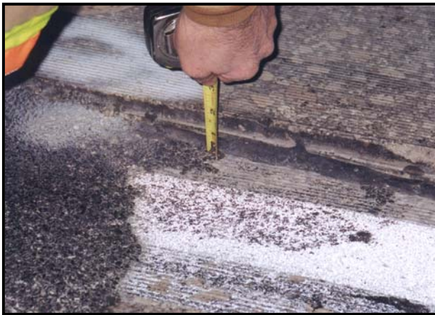
Fig. 4 Bridge approach pavement settlement and damage caused by erosion and construction errors
