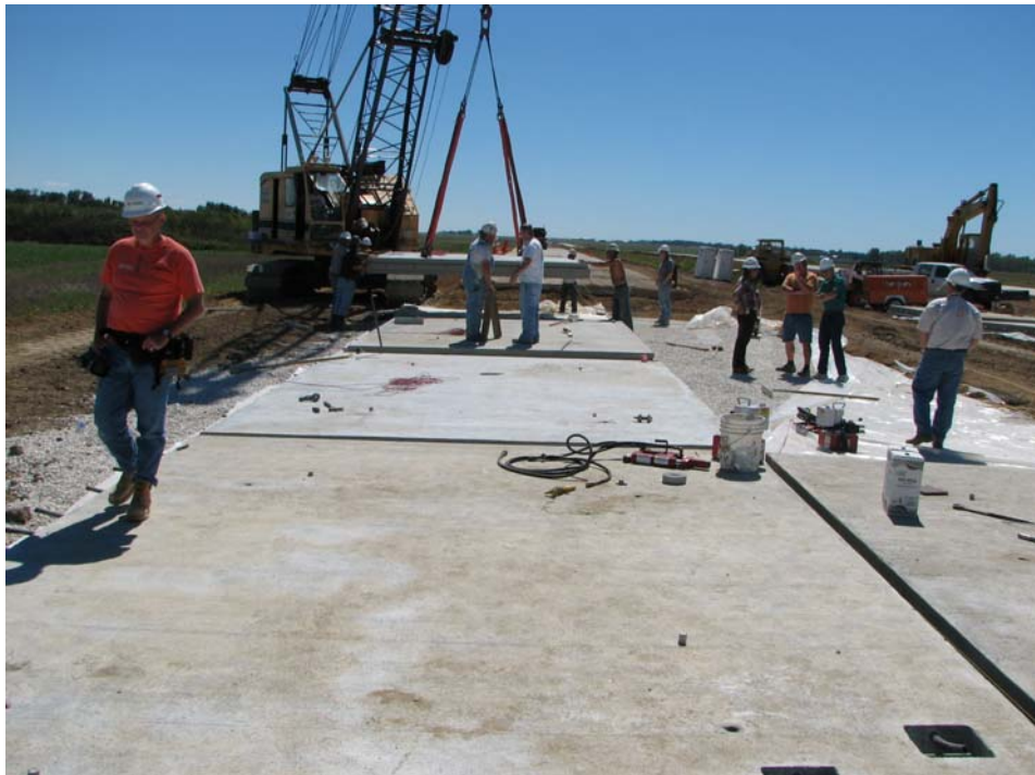
Fig. 10B Keyway with epoxy
