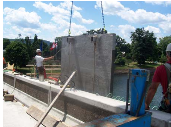
Figure 11: Box Beams with Pockets for Panels Connection Figure 12: Panels Dropped In From Above
