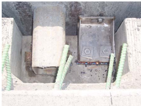
Figure 14: Panel Connection Secured in Pocket.
