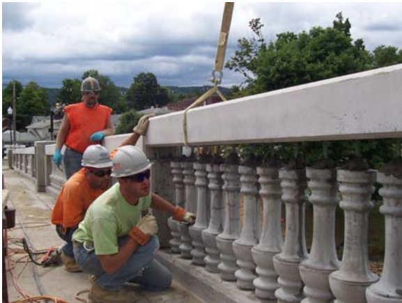
Figure 20: Drop In Of Pre-cast Handrail.
