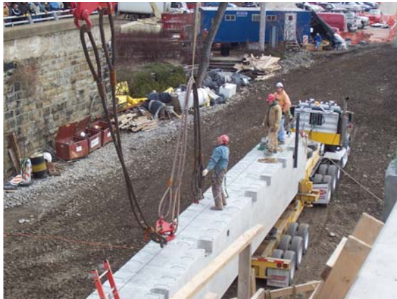
Figure 11: Box Beams with Pockets for Panels Connection Figure 12: Panels Dropped In From Above
