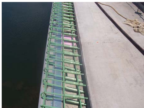
Figure 15: The Two Foot Deck Strip Ready To Be Poured.
