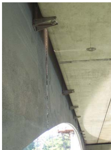
Figure 16: Panels Secured at Bottom of Box Beams.
