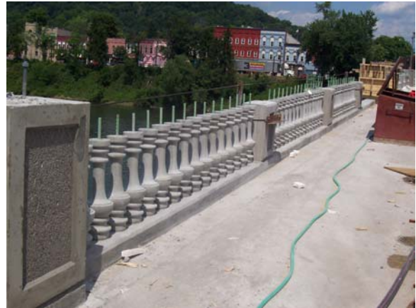
Figure 19: Baluster Grouted In Place.
