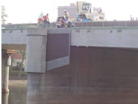
Figure 13: Panels Being Secured Into Pockets.
