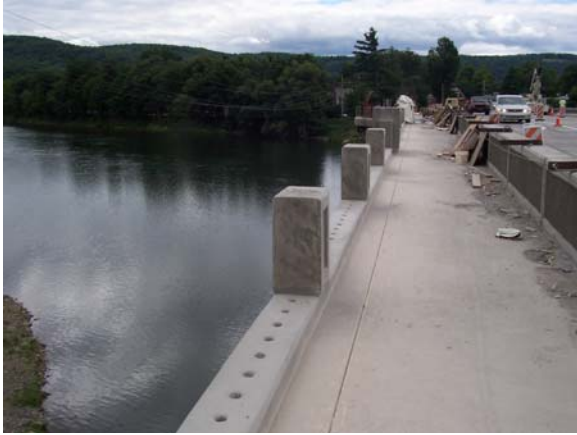
Figure 18: After Deck, Curb and Columns Are In Place.
