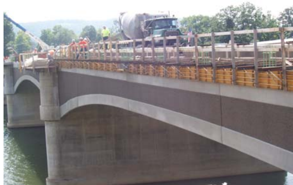
Figure 17: Pouring of Two Foot Deck Strip Over Panels.
