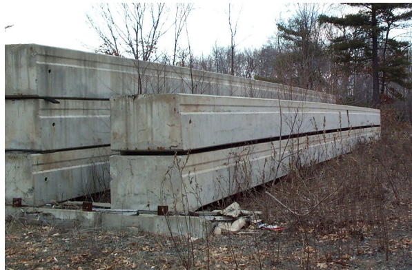
Figure 1: Stockpiles Bridge Beams
