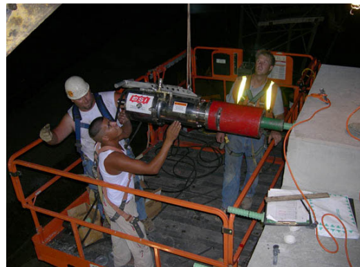
Stressing of post-tensioning bars
