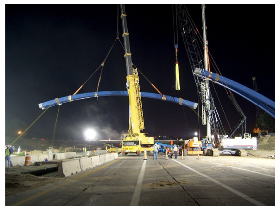
Night time erection of steel arch ribs
