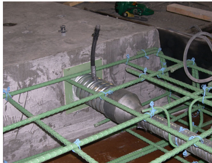
Slab panels were match cast to fit vertical curvature of deck
