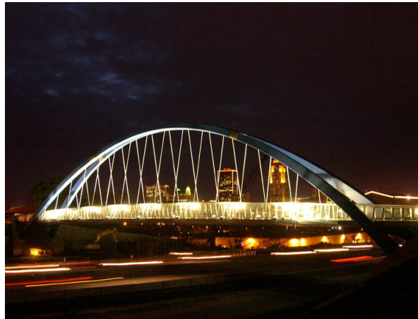
Aesthetic lighting completes the bridge near the Botanical Center
