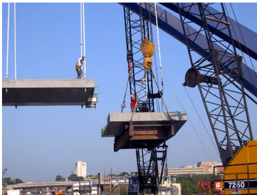
Precast panel lifted in place
