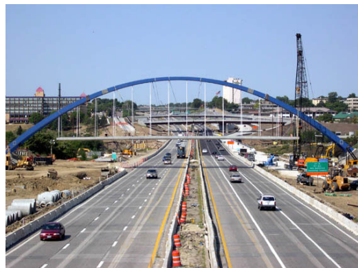
Segmental construction minimized traffic impacts
