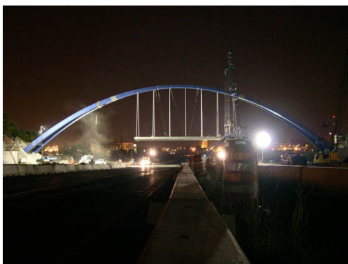
Nighttime erection of precast deck
