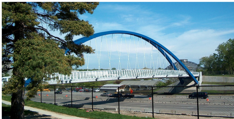
Looking northwest at completed bridge near the Botanical Center
