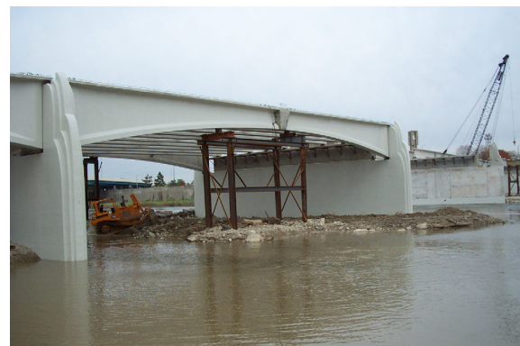
Fig. 5 Temporary shoring supporting fascia girder segments
