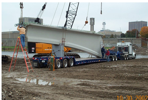
Fig. 4 Transportation of fascia girder segments
