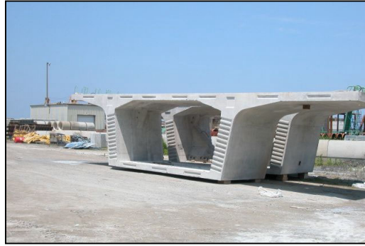
Fig. 2 Precast Approach Span Segment
