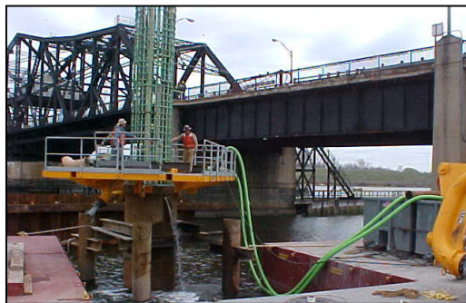
Fig. 4 Drilled Shaft Construction
