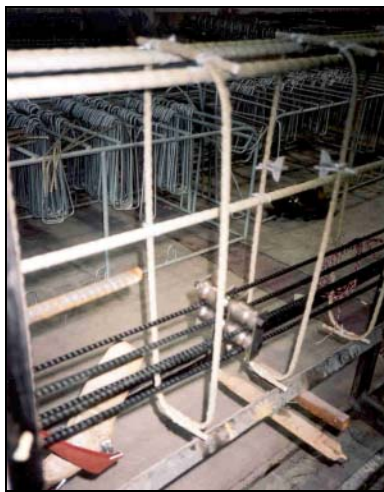
Figure 6. Stirrups (C-shape)
