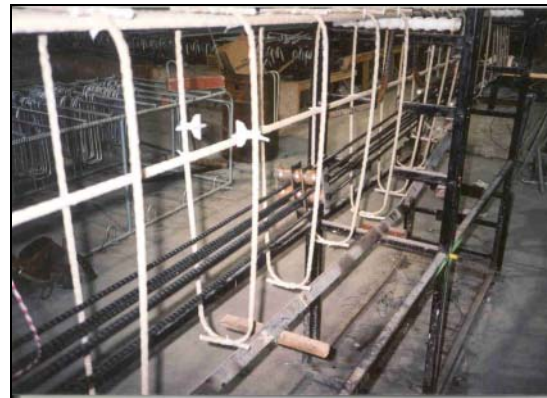
Figure 7. GFRP reinforcement configuration
