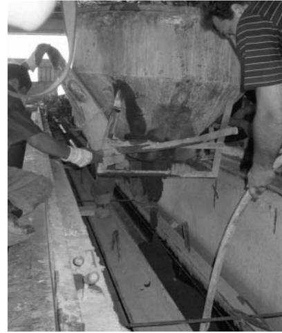
Fig. 10 and Fig. 11 Prepared RPC mix and the process of pouring RPC in the formwork (Pojatno, Croatia, May 2003)
