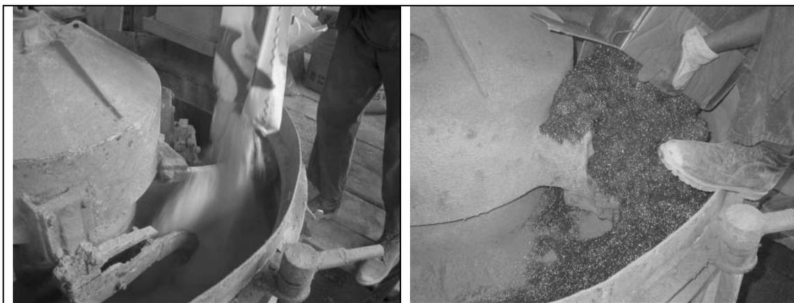
Fig. 8 and Fig. 9 Adding RPC components to the mixer (Pojatno, Croatia, May 2003)
