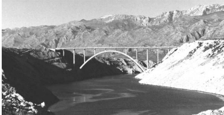
Fig. 1 Maslenica Bridge, concrete arch 200m in span, Croatia, 1997, Author: J. Radic [2]
