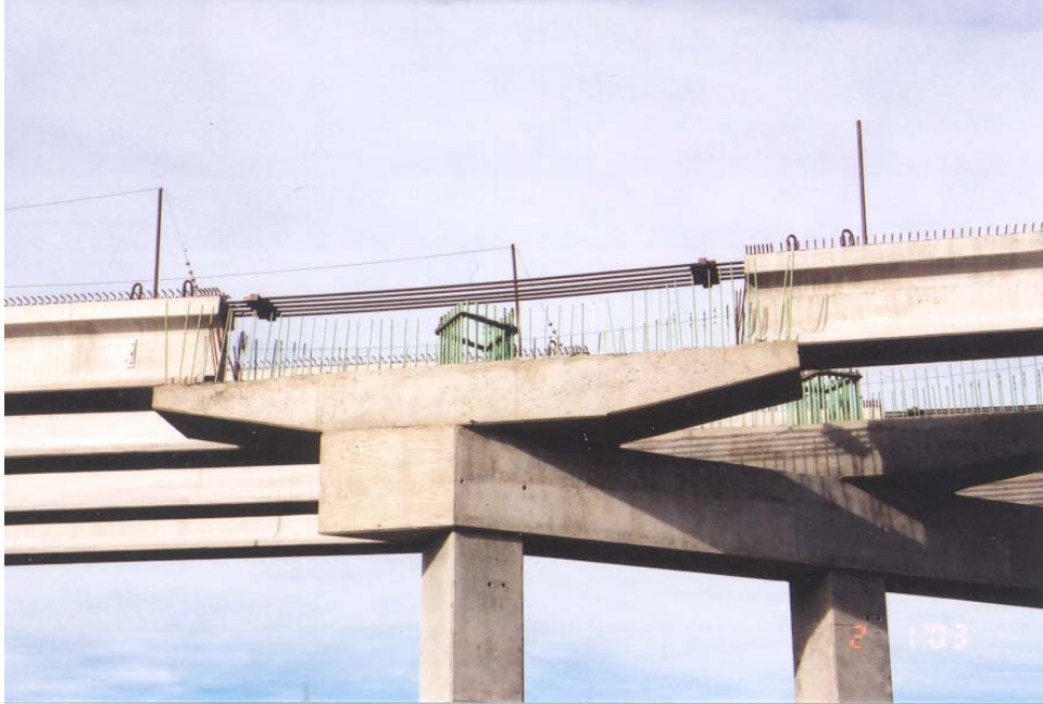
Fig. 2 Showing the pier section before placement of the pier blocks.
