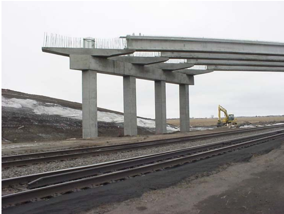
Fig. 1 Precast girders seated over the CIP haunched beam
