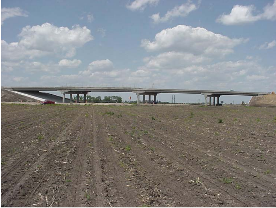
Fig. 5 Completion of bridge construction
