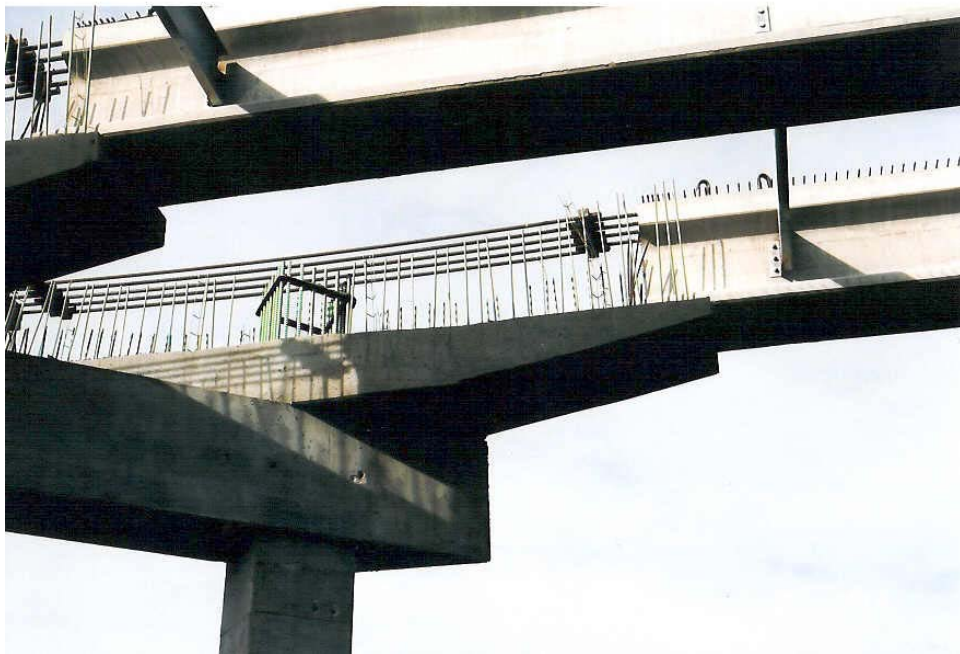
Fig. 3 Close-up view of the continuity connection
