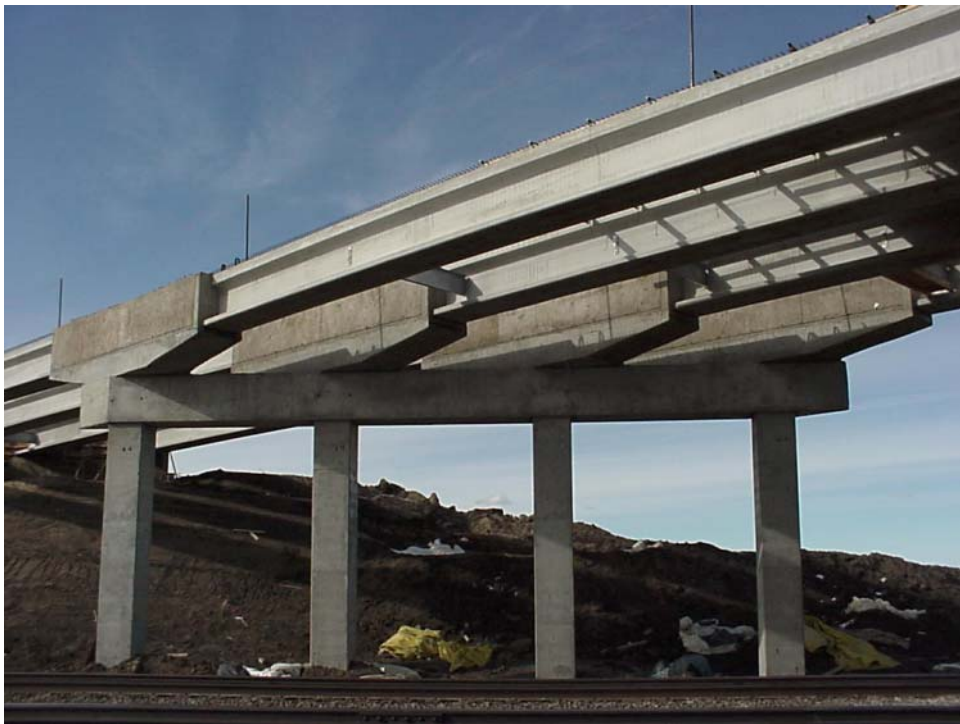
Fig. 4 Girder continuity by placing the pier block
