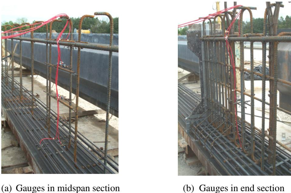
Fig. 5 Instrumented Prestressed Concrete Beams
