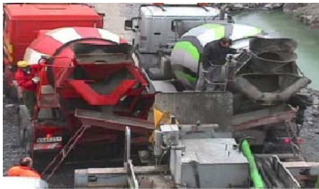
Fig. 8 Arrangement for continuous discharge
