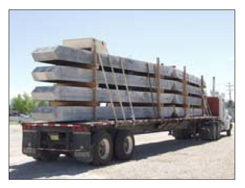
Fig. 8 Trucking eight panels per truck
