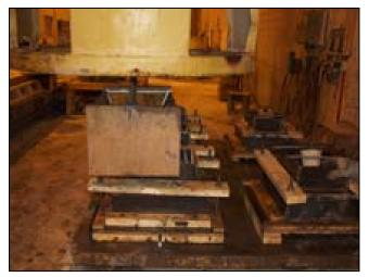
Fig. 19 Casting the anchor blocks
