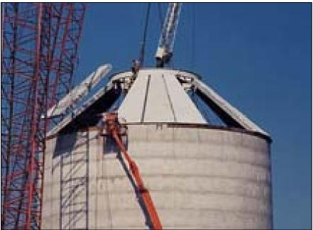
Fig. 10 Flying panels into place using a mobile crane
