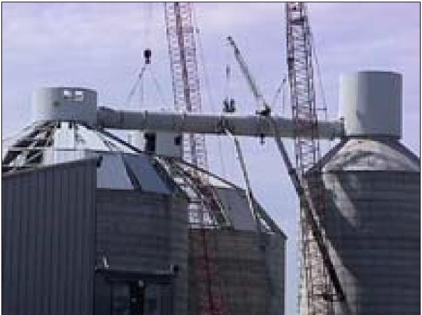
Fig. 12 All 3 clinker silos and connecting feeder conveyors. (Precast roof at right)
