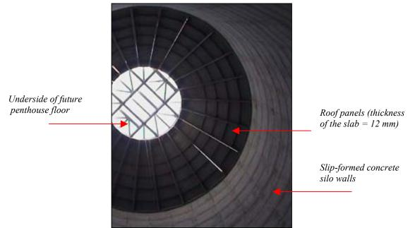
Fig. 11 View from underside, looking up at panels
