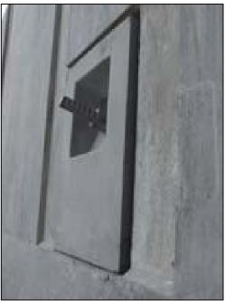
Fig. 22 Anchor plate installed, elevation view
