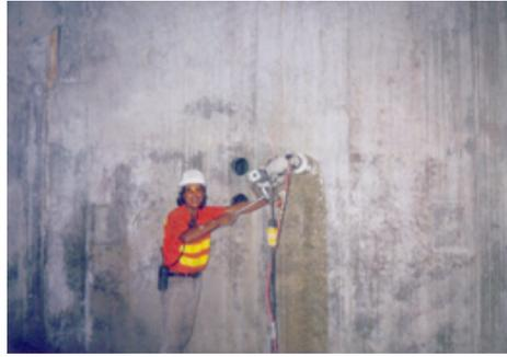
Fig. 4 Core driller removing cores from cells.
