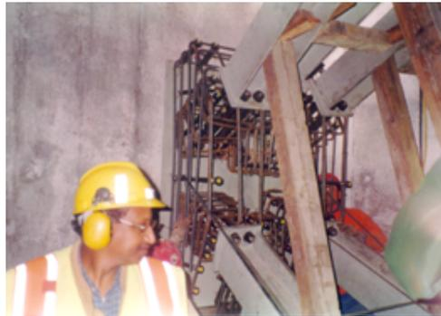
Fig. 6 Spider anchors are assembled inside the pontoon cells.
