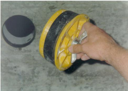
Fig. 5A Watertight plugs are installed in the core holes maintaining integrity.
