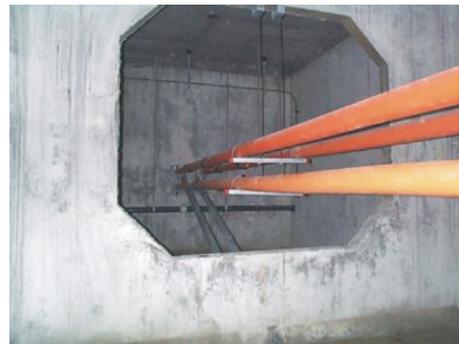
Fig. 5B Post-tensioning tendons run through the pontoon cells.
