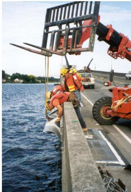
Fig. 8 Installation of wave deflectors.
