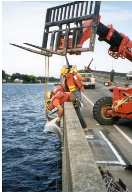
Fig. 8 Installation of wave deflectors.
