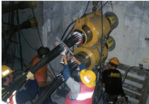
Fig. 7 Post-tensioning operations with 24 feet of elongation.
