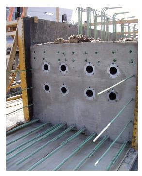
*Fig.* 7 – *Post tensioning bridge plates at end of longitudinal girder frame blockout.*
