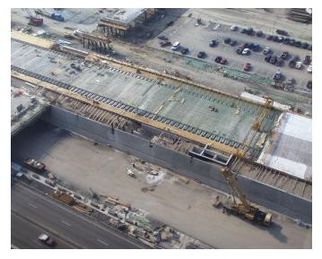
Fig. 12 – Floorbeams erected awaiting deck slab casting
