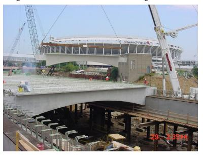
Fig. 11 - Floor beam erection
