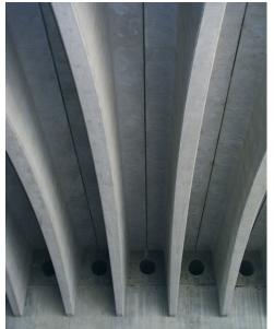
Fig. 8 – Detail of floorbeams at connection to longitudinal girder. Note holes in diaphragm for ventilation system.
