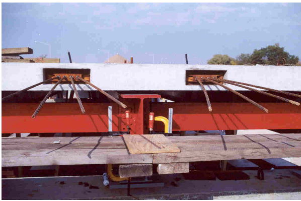
Fig. 11 Post-tensioning of 4(0.6 in.) strands
