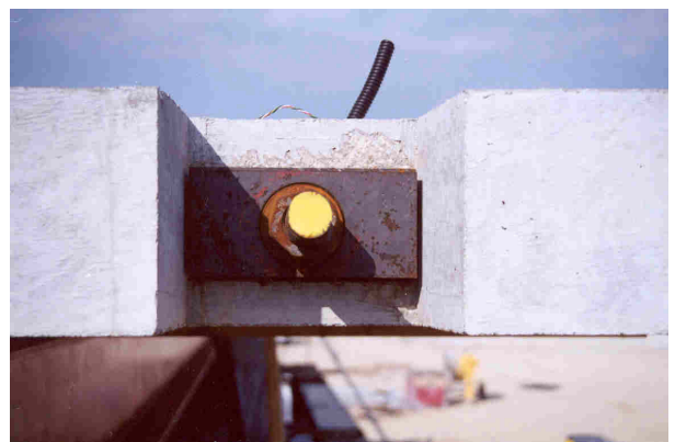
Fig. 12 Post-tensioning of Dywidag bar
