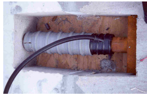
Fig. 17 Coupling of Dywidag Thread bars
