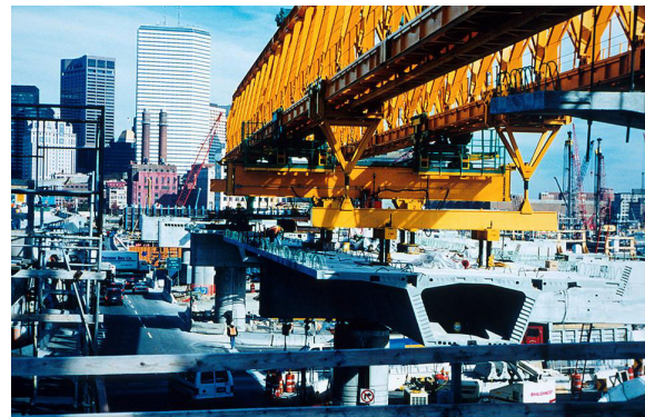
Fig. 6: Balanced cantilever erection using a gantry
