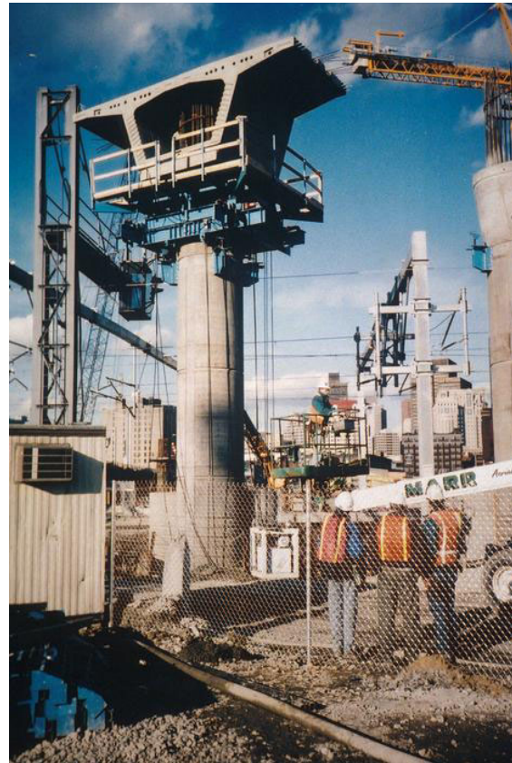
Fig. 9: Precast fixed segment in place on support frame
