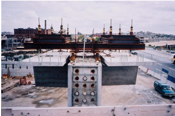
Fig. 12: Saw cut segments being erected
