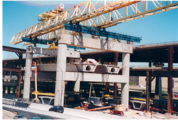
Fig. 7: Span-by-span erection at double-deck bents with overhead gantry
