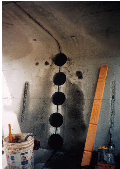
Fig. 11: Coring of shear keys
