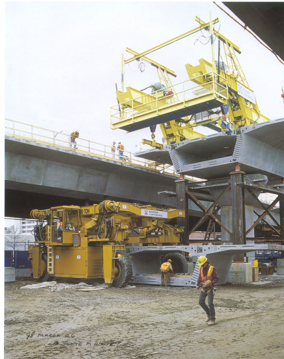
Fig. 5: Beam and winch erection of segment; low headroom segment transporter
