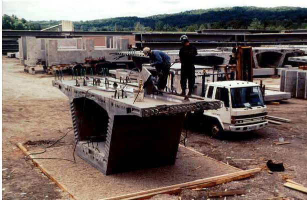
Fig. 10: Saw cutting of segment
