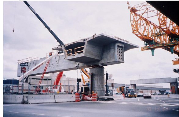
Fig. 13: Straddle bent with precast segments
