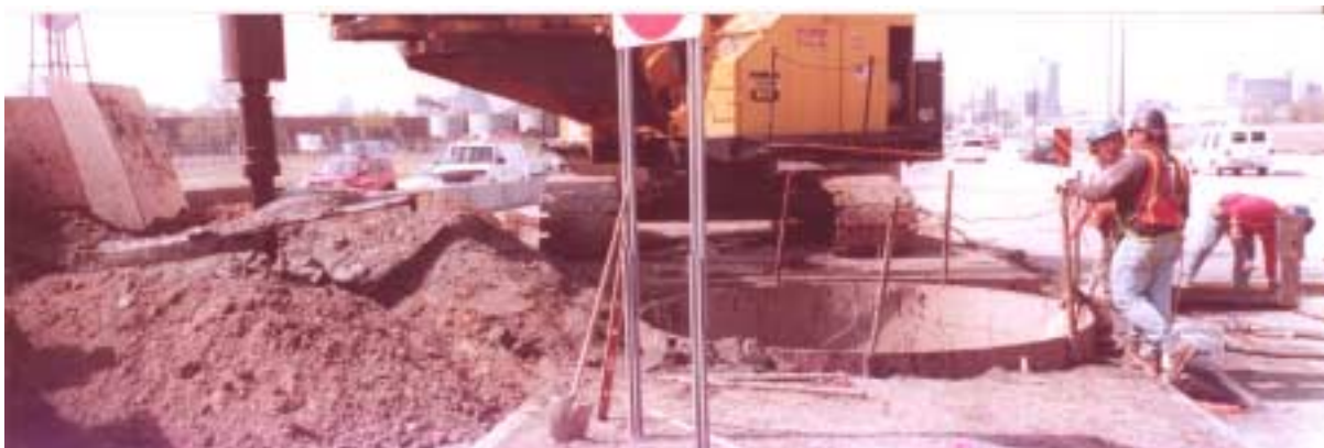
Drilled Caisson in Median of Hiawatha Avenue (TH-55)
