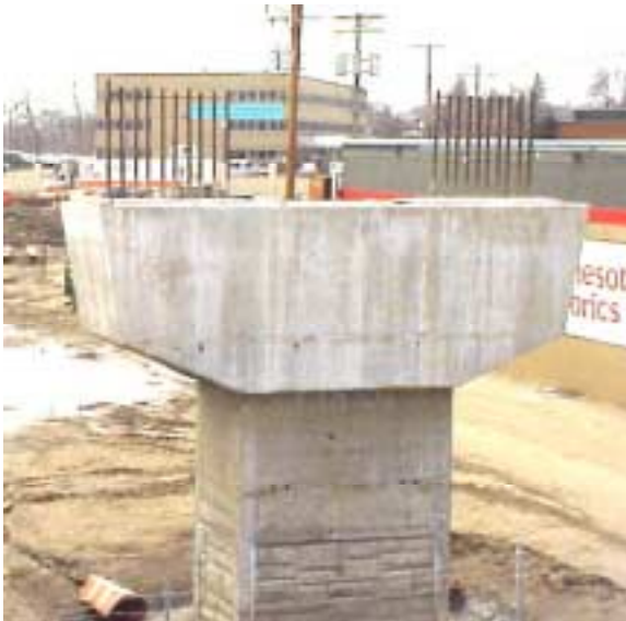
Hinge Reinforcement at Pier
