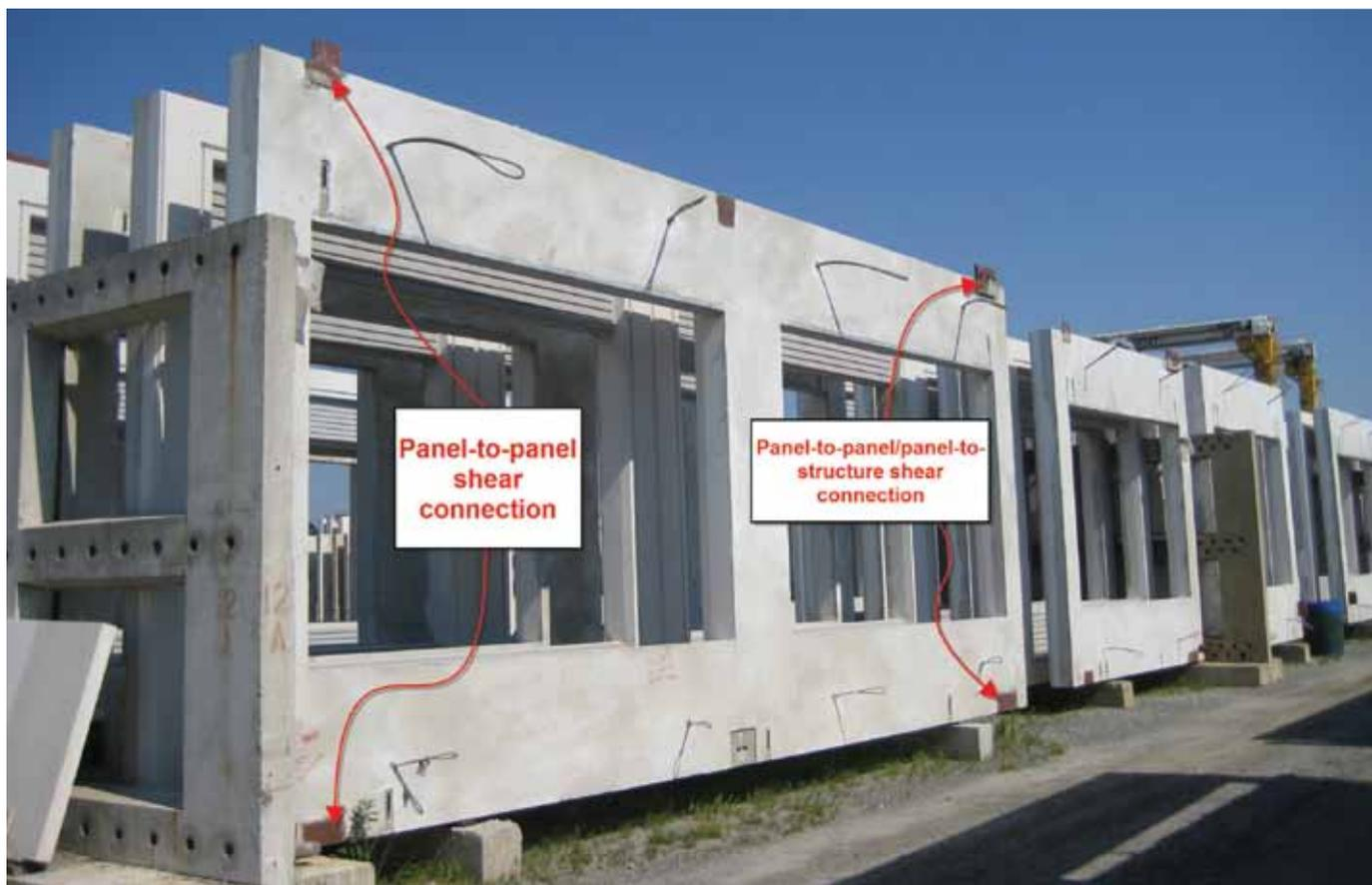
Figure 4. Rear elevation of a typical panel in storage. Figure 5 shows the connection details.
