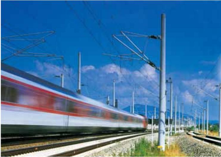
Concrete poles support overhead catenary wires for high-speed rail. Photo courtesy of Valmont Industries, Inc.
