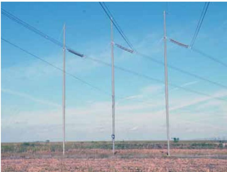
Reverse tapered spun concrete poles also allow for taller poles and lighter weight. In addition to the improved aesthetics, the construction allows for direct embedment in the soil and results in reduced transportation and installation costs. Photo courtesy of Valmont Industries, Inc.
