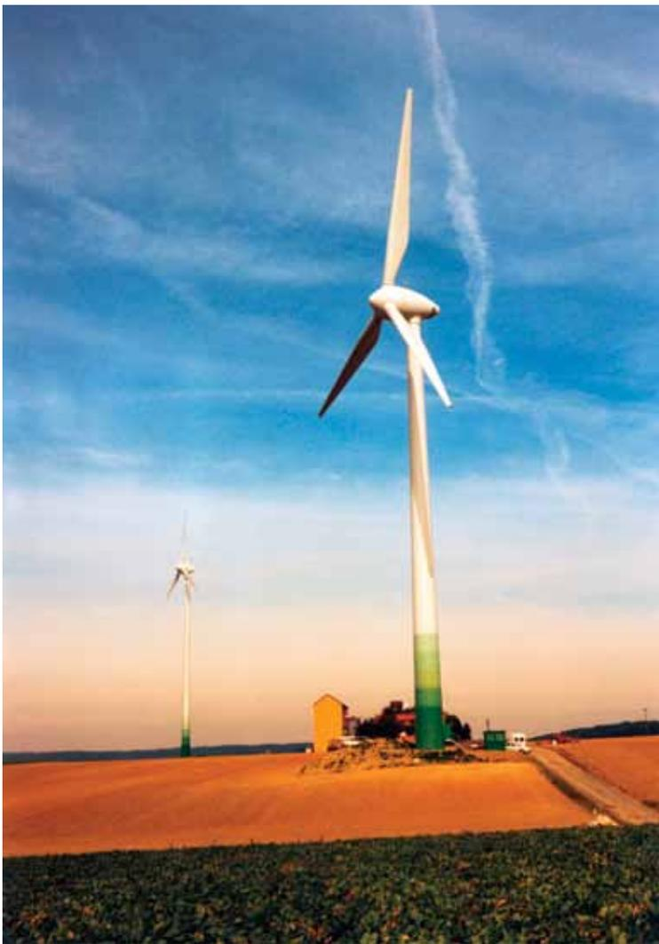
Wind turbines up to 1.2 MW in capacity have been supported on concrete poles in northern Europe. Future improvements in wind-turbine technology, coupled with anticipated increases in oil prices and public concern over pollution from burning fossil fuels, may result in the spread of wind farms and, hence, the need for large concrete poles to support the massive turbines. Photo courtesy of Valmont Industries, Inc.
