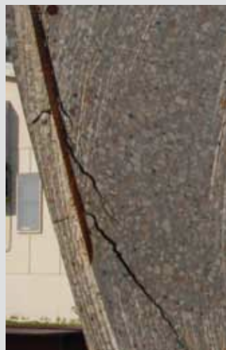
Debonding of the reinforcement
