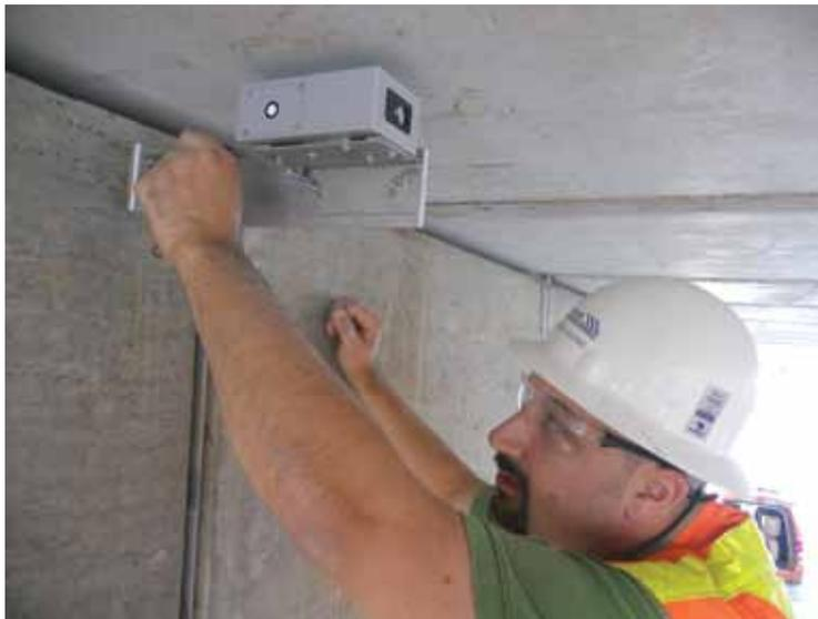
Jaimy Juliano adjusts a laser for long-term monitoring of deflections on the Pembroke Bridge. This type of laser technology was first used to monitor instantaneous out-of-plane deflections to prevent buckling of members being installed in the Huey P. Long Bridge in Louisiana. **Photo courtesy of Applied Geomechanics.**
