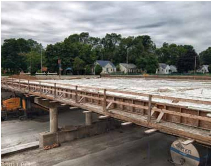
The cast-in-place concrete deck of the Pembroke Bridge in Southfield, Mich., is curing. Photo courtesy of Paul Grigonis.
