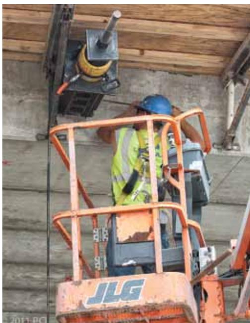
The second post-tensioning of the carbon-fiber-composite cable places the cast-in-place concrete deck of the Pembroke Bridge in compression. Photo courtesy of Paul Grigonis.
