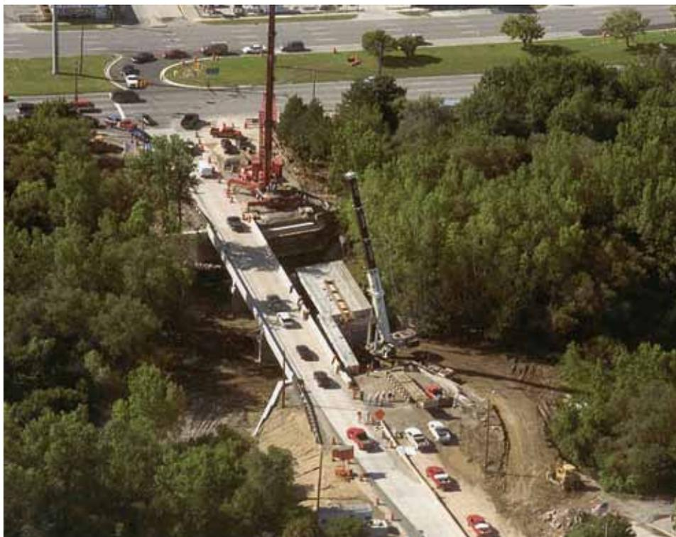
The Bridge Street Bridge in Southfield, Mich., completed in 2001, was the first bridge in the United States to use carbon-fiber-reinforced polymer (CFRP) reinforcement, CFRP pretensioning tendons, and carbon-fiber-composite cable post-tensioning throughout. Monitoring of this bridge will continue until 2020, providing long-term data on its performance. **Photo courtesy of Nabil Grace.**
